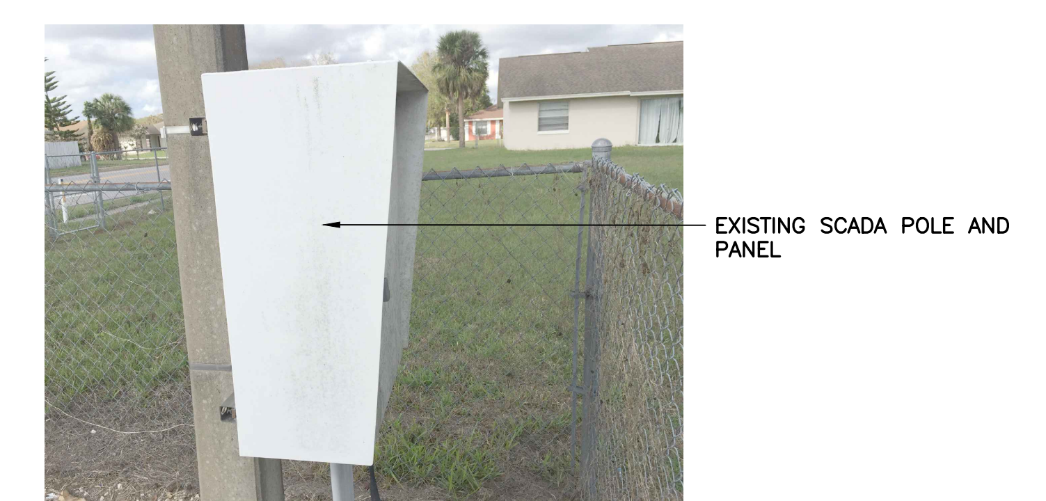
PUMP STATION 3283 FIGURE NO. 2
