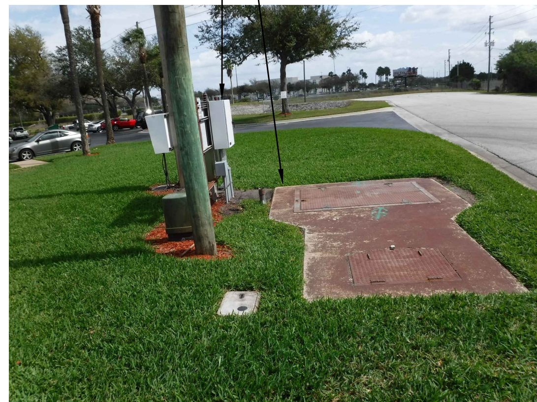
EX. PUMP STATION SITE
