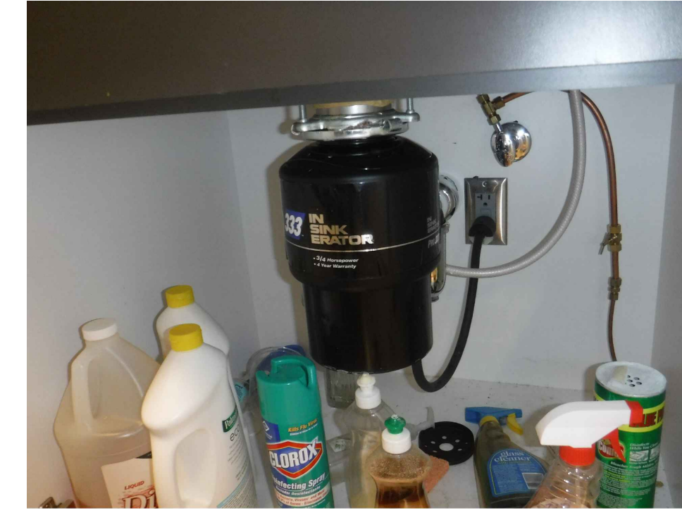
EXISTING DISPOSAL TO BE REMOVED AND REINSTALLED
