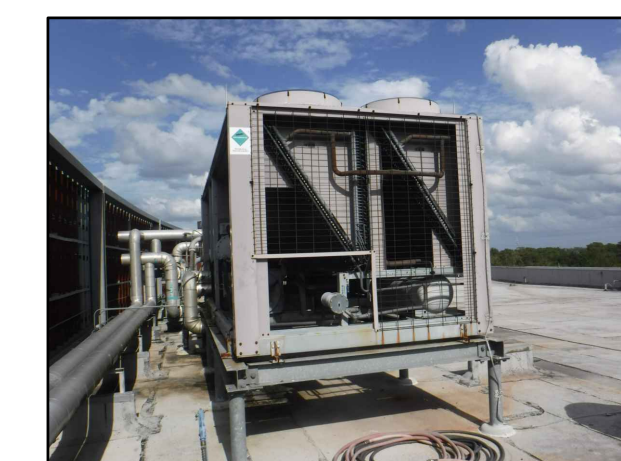
EXISTING LIGHTNING PROTECTION CABLING AND AIR TERMINALS TO BE REMOVED AND REINSTALLED
