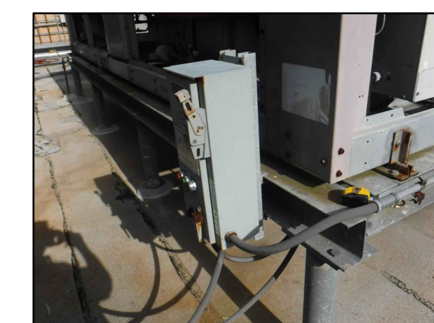
EXISTING DISCONNECT TO BE REMOVED AND REINSTALLED
