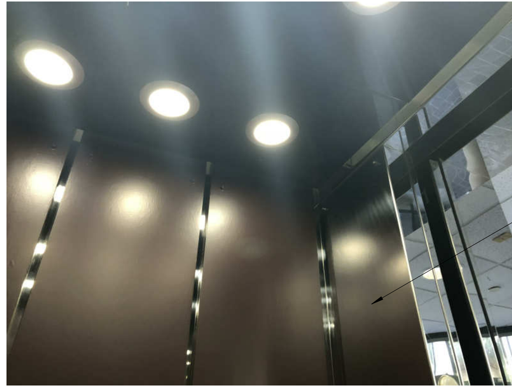
RETURN PANEL - RE-CLAD IN MIRROR STAINLESS AND PROVIDE OUT-OUTS FOR SIGNAL AND OPERATING FIXTURES. SEE SPECIFICATIONS FOR ADDITIONAL INFORMATION
