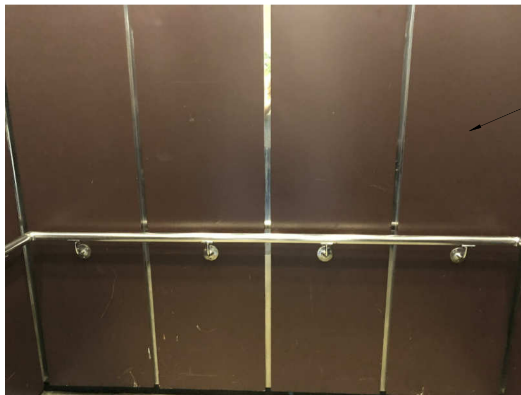
WALL PANELS - FLAT LAMINATE - STANDARD WILSONART - COLOR AND PATTERN TO BE SELECTED UPON SUBMITTAL. SEE SPECIFICATIONS FOR ADDITIONAL INFORMATION
