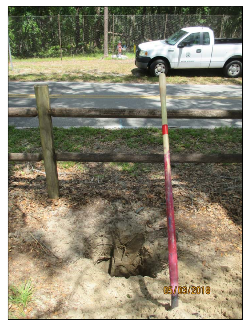
WATER LINE EXCAVATION PHOTO NO. 1 (ONSITE)
