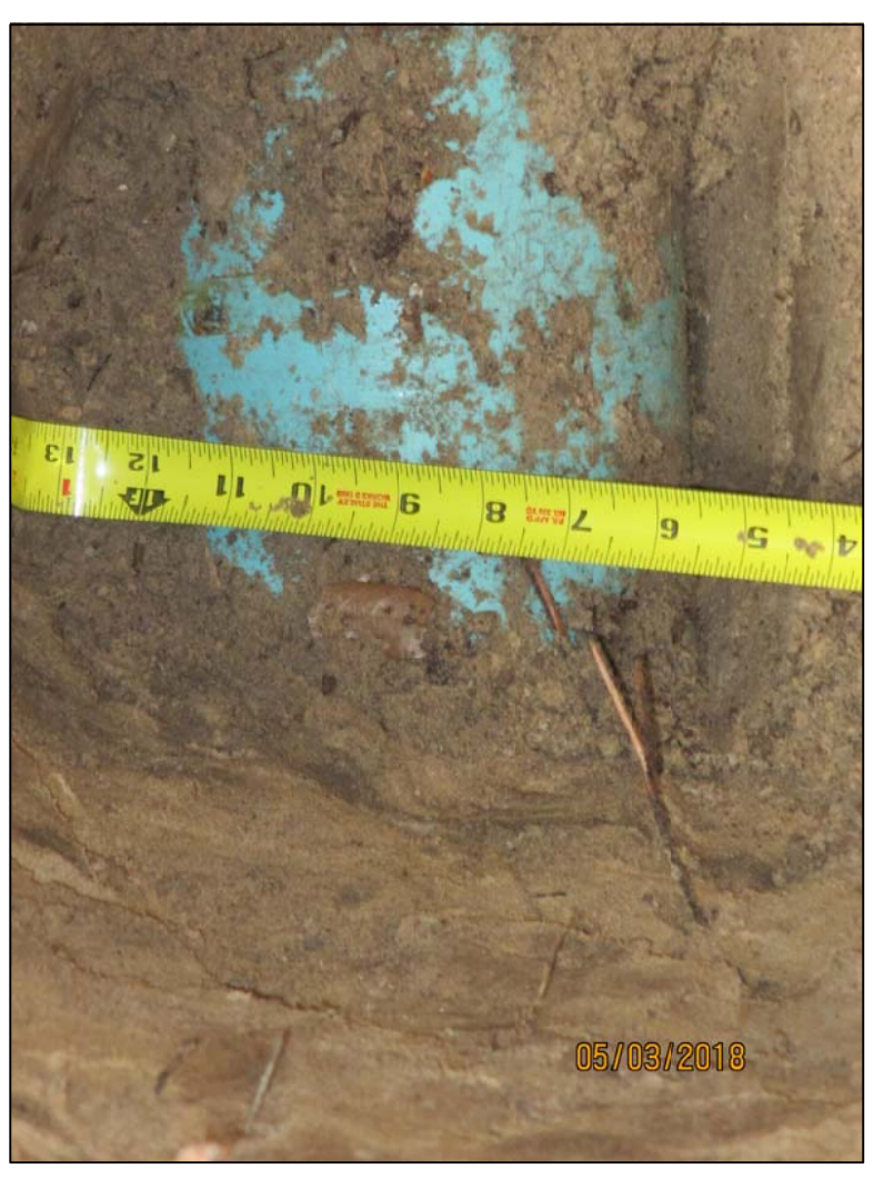
WATER LINE EXCAVATION PHOTO NO. 3
