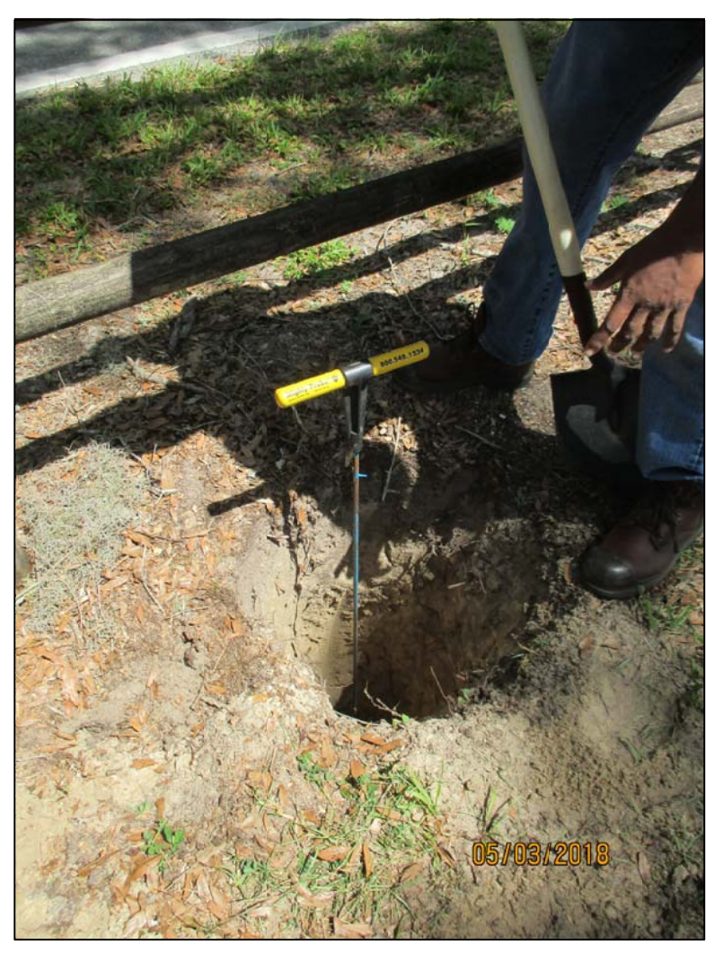
WATER LINE EXCAVATION PHOTO NO. 2
