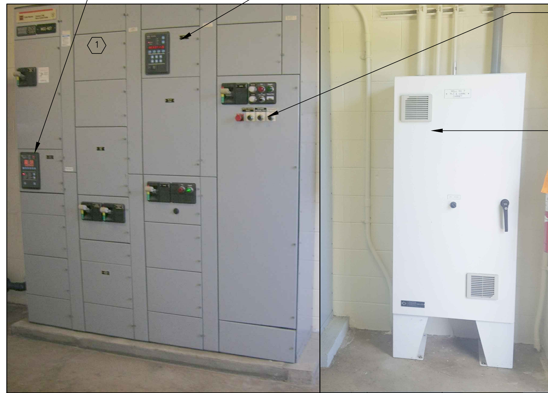
EXISTING WELL NO.7 MCC NOT TO SCALE
