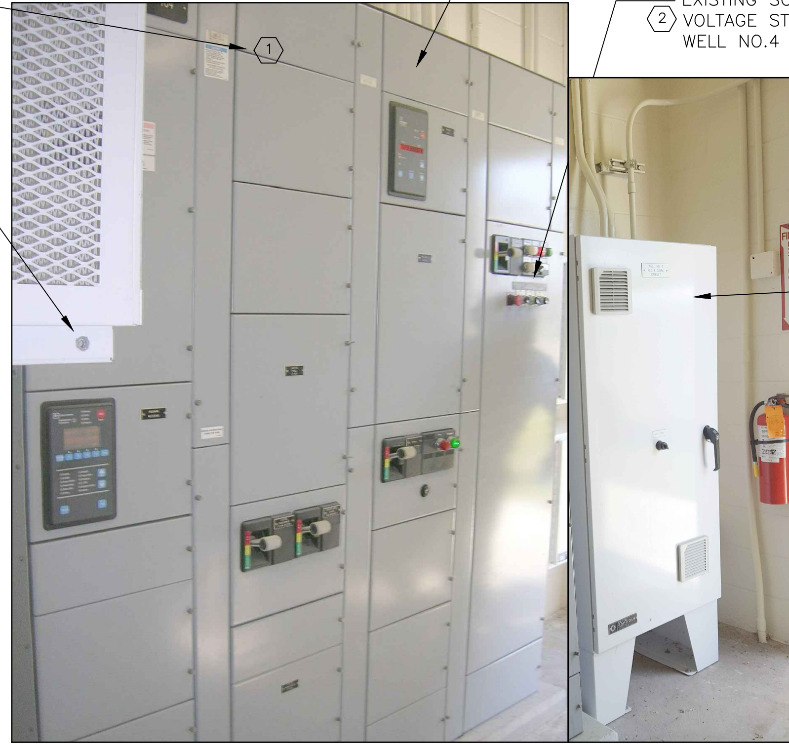
EXISTING WELL NO.4 MCC NOT TO SCALE
