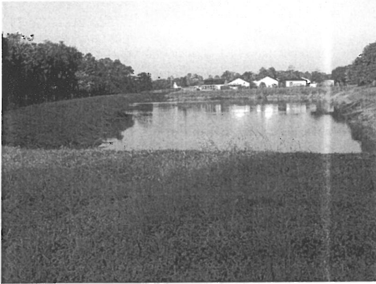
POND 6953- DEAN ROAD, SOUTH OF CARMEL PARK DRIVE, TRACT 6027 LANDS DESCRIBED IN OFFICIAL RECORDS BOOK 4164, PAGE 2542 ORANGE COUNTY, FLORIDA
