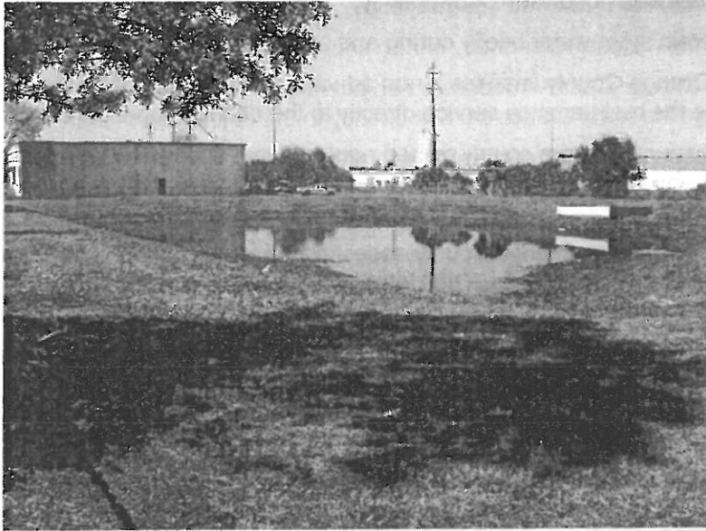
POND 6239- EDGEWATER DRIVE/ ALL AMERICAN BOULEVARD, SOUTH OF EDGEWATER DRIVE, LOTS 19 AND 20, AMERICAN BUSINESS CENTER, AS RECORDED IN PLAT BOOK 8, PAGES 21 AND 22, ORANGE COUNTY, FLORIDA
