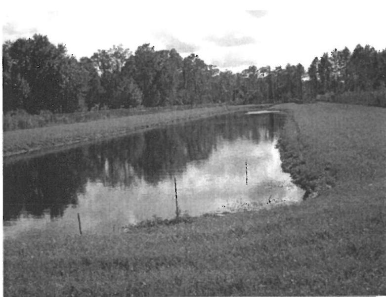
POND 0079- ROCK SPRINGS ROAD, NORTH OF LESTER ROAD LANDS DESCRIBED IN OFFICIAL RECORDS BOOK 5827, PAGE 1865 ORANGE COUNTY, FLORIDA
