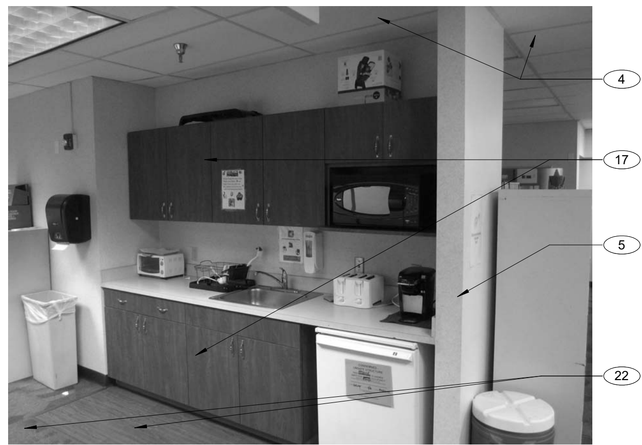
E3 AD230 DEMOLITION IMAGE SCALE: 12" = 1'-0"
