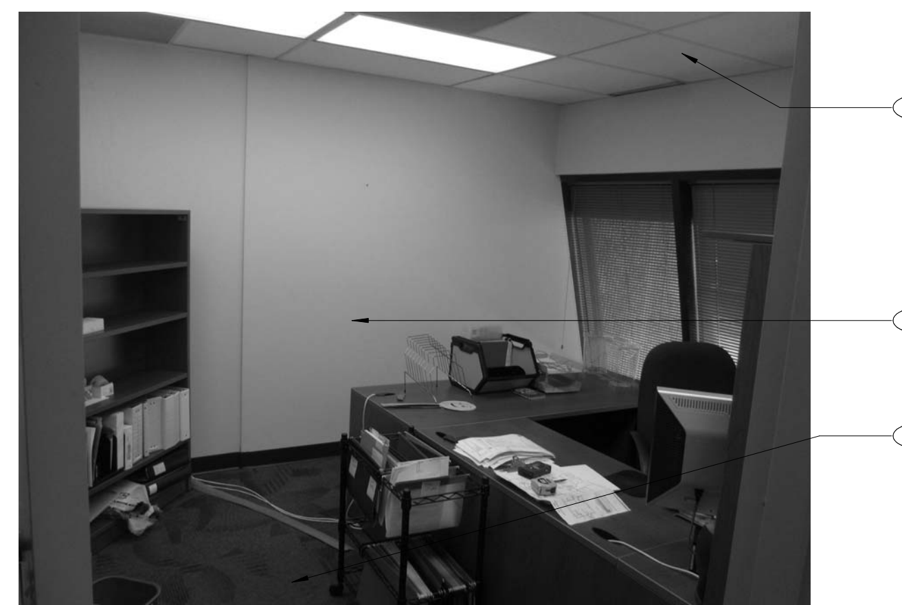
E7 AD230 DEMOLITION IMAGE SCALE: 12" = 1'-0"
