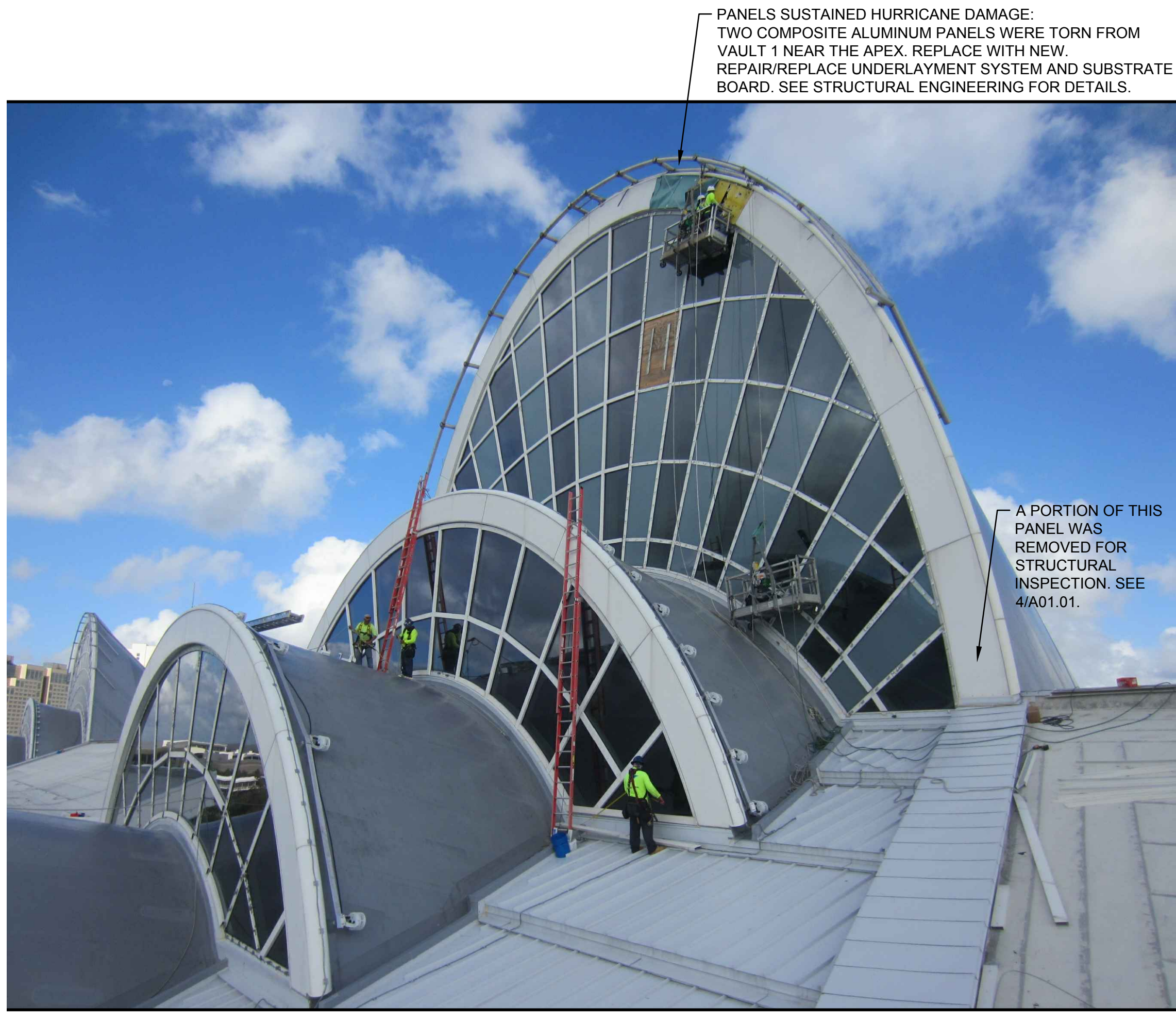
3 PHOTO - SOUTH B - VAULT 1 EASTERNMOST VAULT ON THE SOUTH BUILDING NTS
