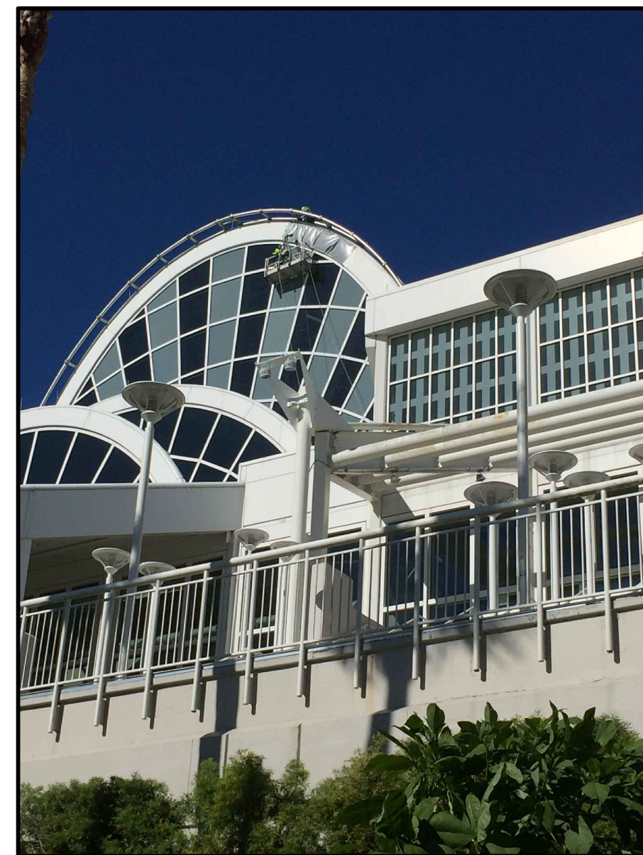
3 SOUTH BUILDING - EAST VAULT OR SOUTH B A01.01 VIEW LOOKING NORTH NTS
