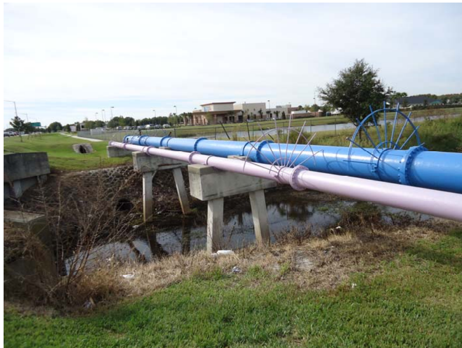
Photo-2: Pipe Crossing at Sky Lake Canal
