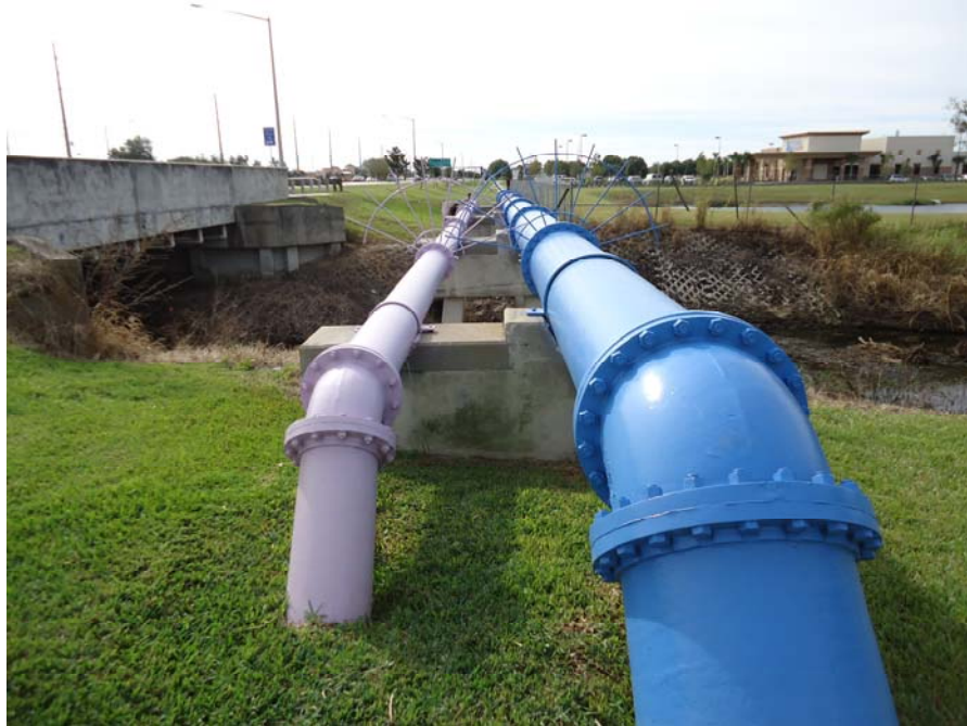
Photo-1: Pipe Crossing at Sky Lake Canal
