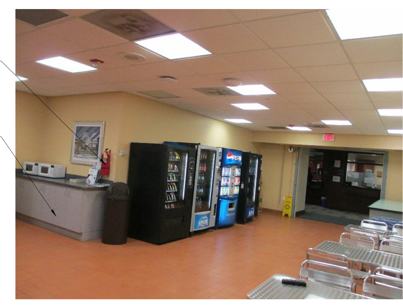
E3 AD102 DEMOLITION IMAGE 06 SCALE: 3" = 1'-0"
