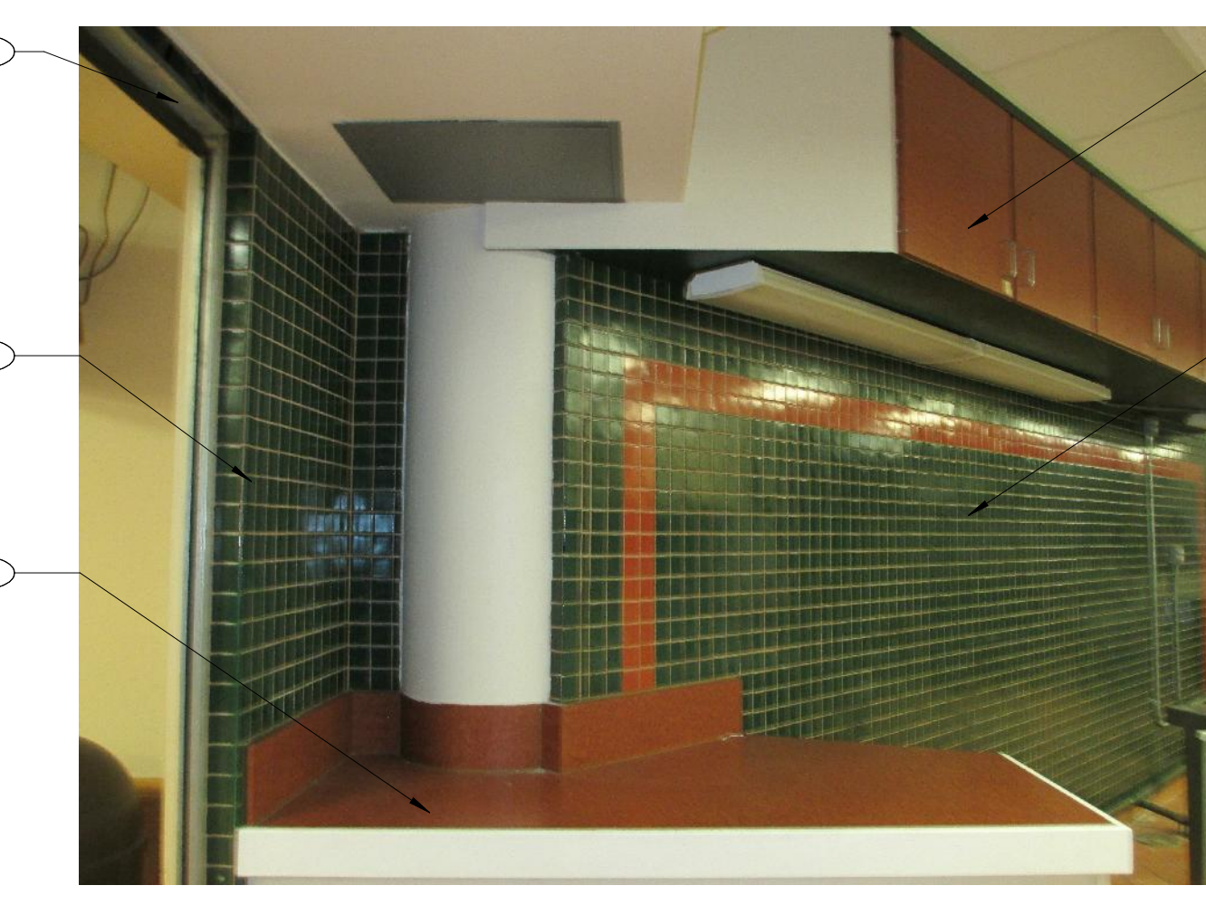
C5 AD102 DEMOLITION IMAGE 11 SCALE: 3" = 1'-0"
