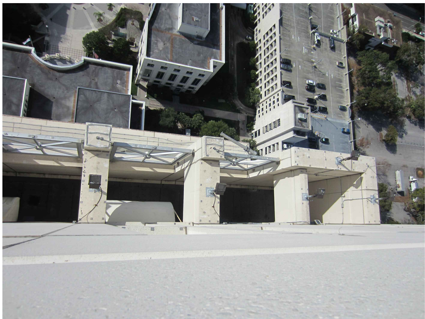
04 LEVEL 23 AERIAL VIEW
