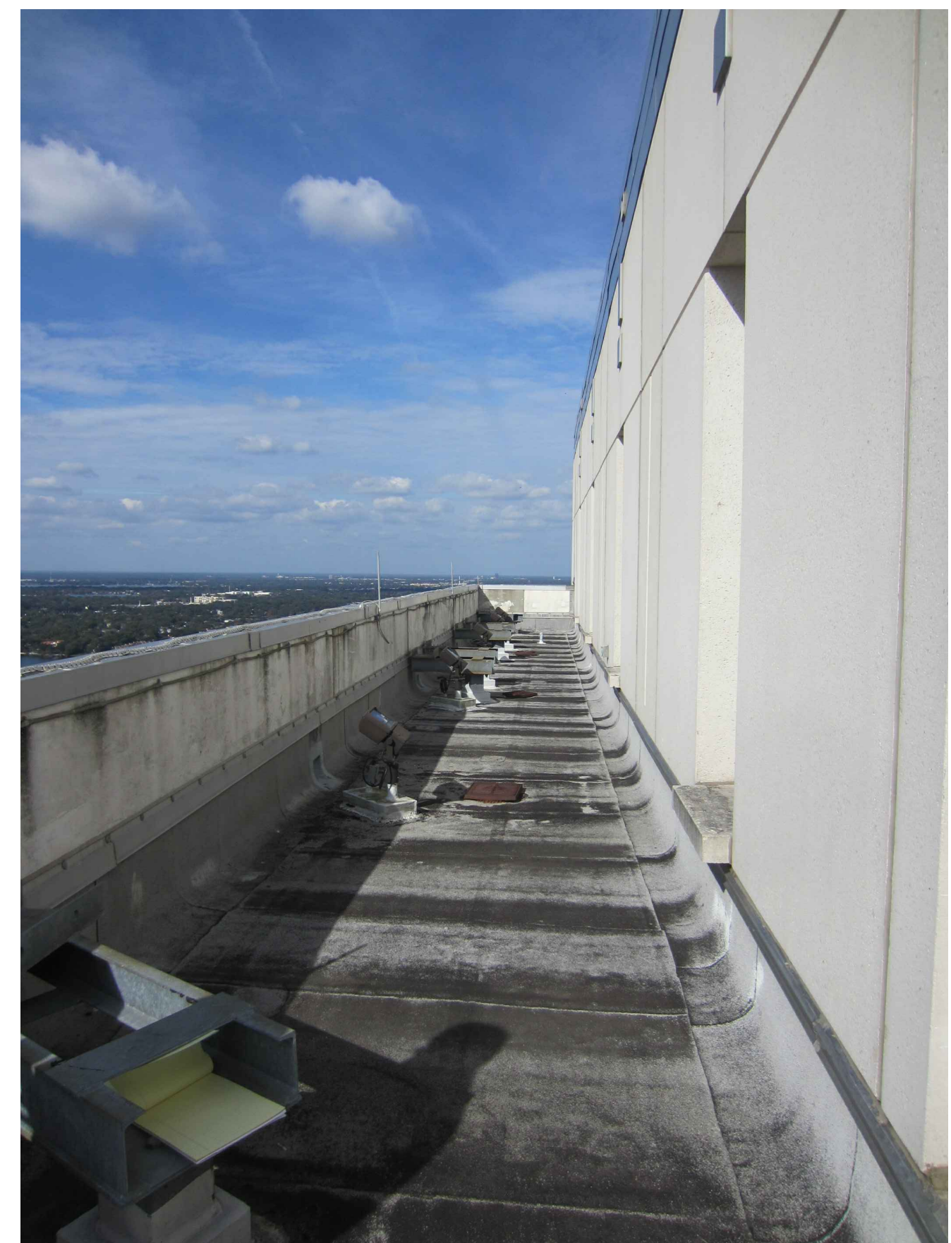
06 LEVEL 24 1/2 SAME LEVEL VIEW
