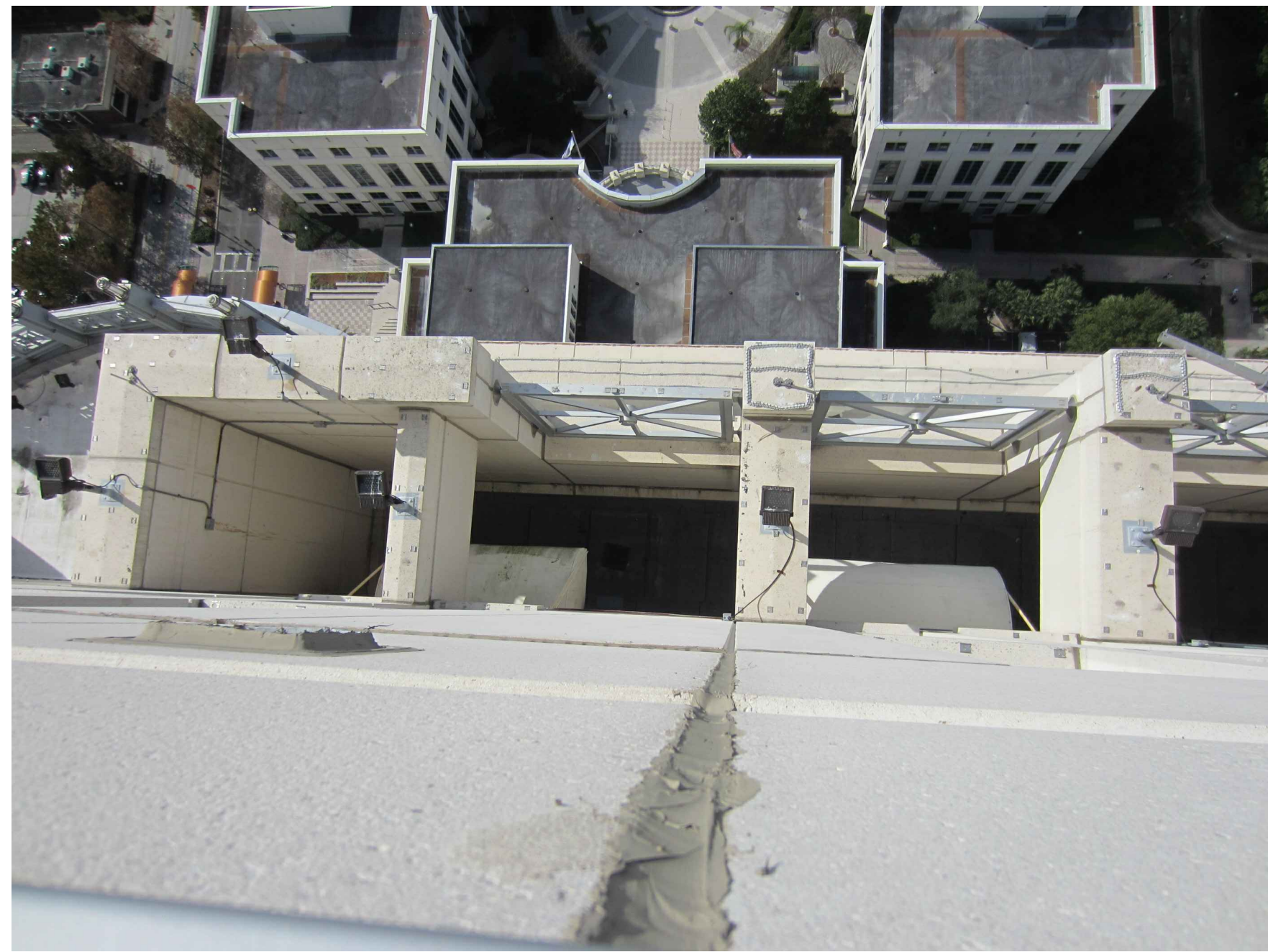
03 LEVEL 23 AERIAL VIEW
