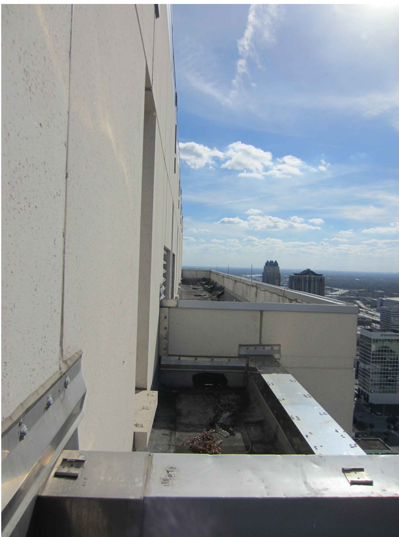
05 LEVEL 24 1/2 SAME LEVEL VIEW
