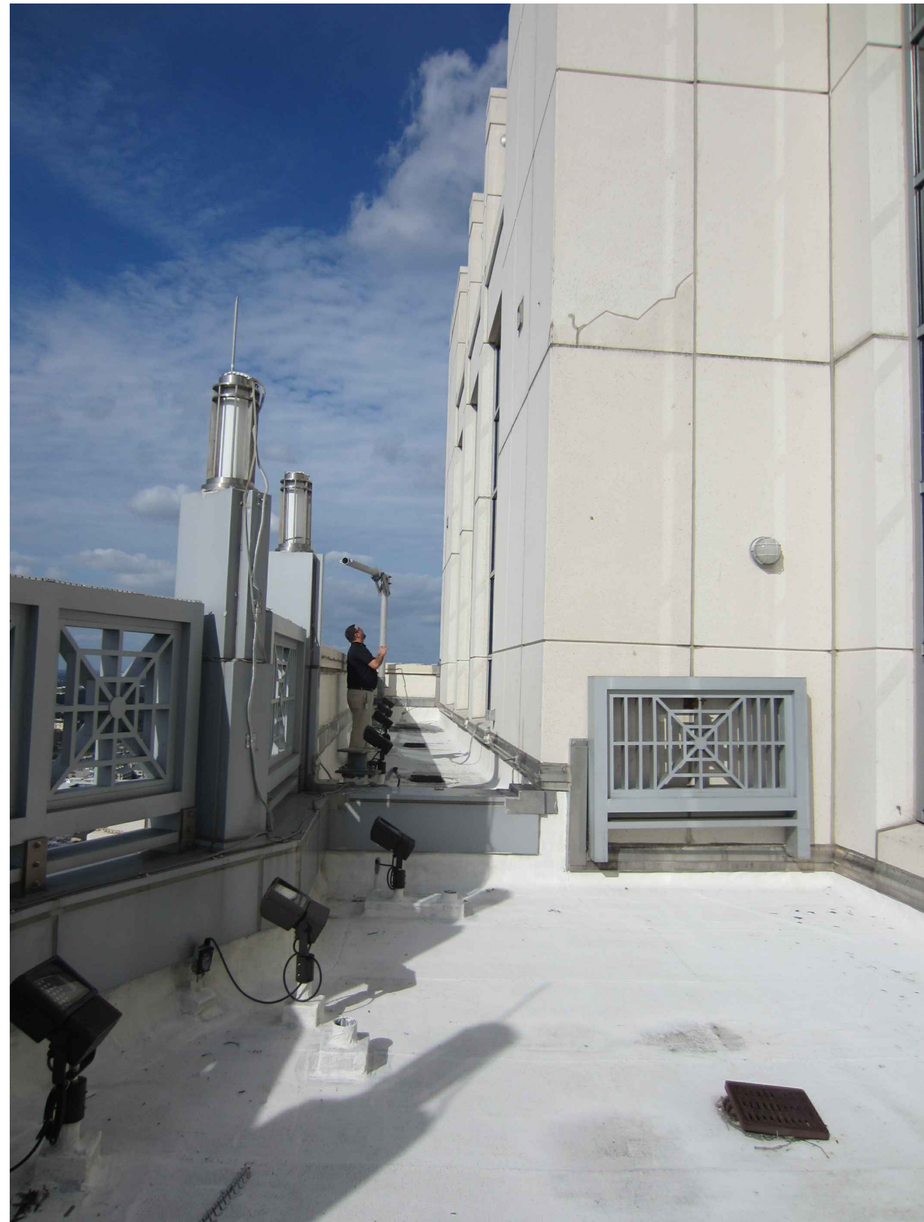
01 LEVEL 21 SAME LEVEL VIEW
