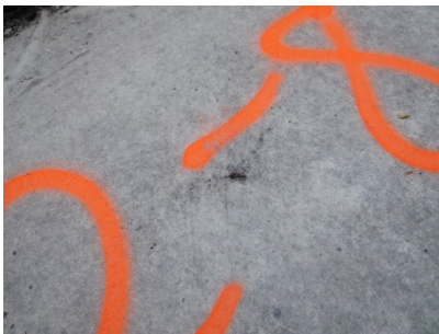
Visual image hole in roof
