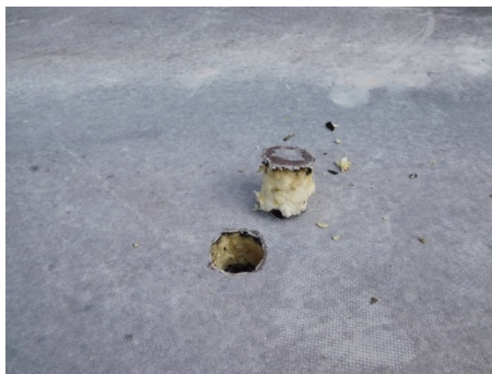
Visual image of wet core cut
