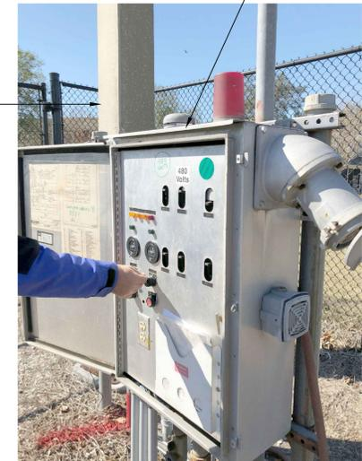
EXISTING PUMP CONTROL PANEL TO BE DISCONNECTED, REMOVED AND RETURNED TO OWNER
