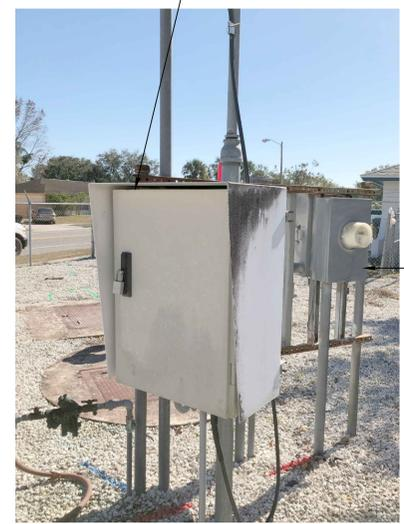
EXISTING UTILITY METER TO BE DISCONNECTED AND REMOVED
