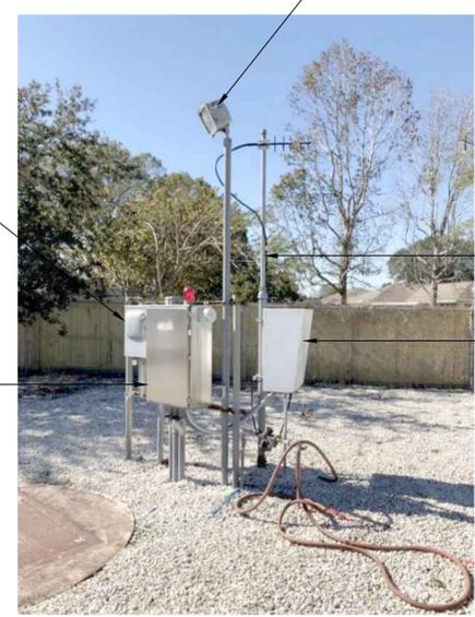
EXISTING MAIN DISCONNECT TO BE DISCONNECTED AND REMOVED
