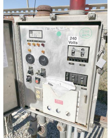
EXISTING PUMP CONTROL PANEL TO BE DISCONNECTED, REMOVED AND RETURNED TO OWNER
