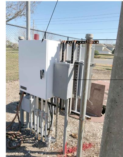
EXISTING SCADA PANEL TO BE DISCONNECTED, REMOVED AND RETURNED TO OWNER
