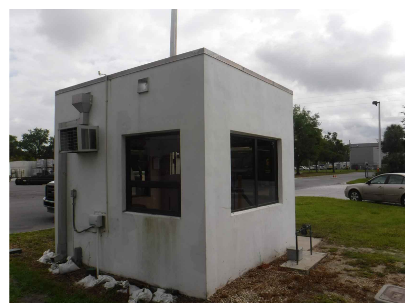
EXISTING GUARD SHACK (NORTH)
