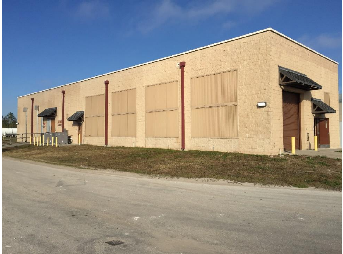
Figure 3.10 Existing Generator/Electrical Building
