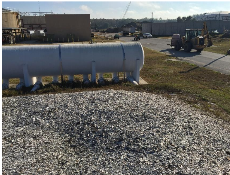
Figure 3.13 Existing Biofilter - View from West
