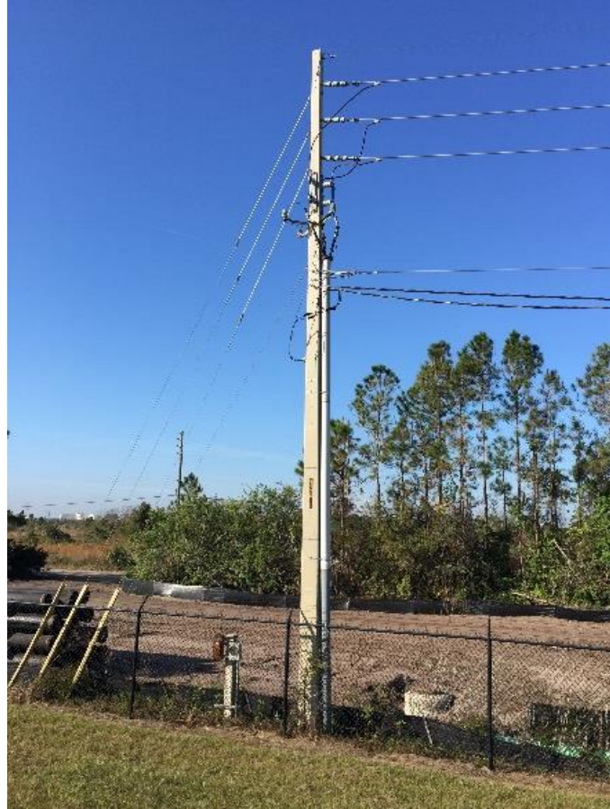
Figure 2.1 OUC Service Drop "A" West Property Line
