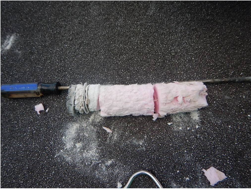
Photo 1 – 6" Insulation Core Sample at Lower Roof Area
