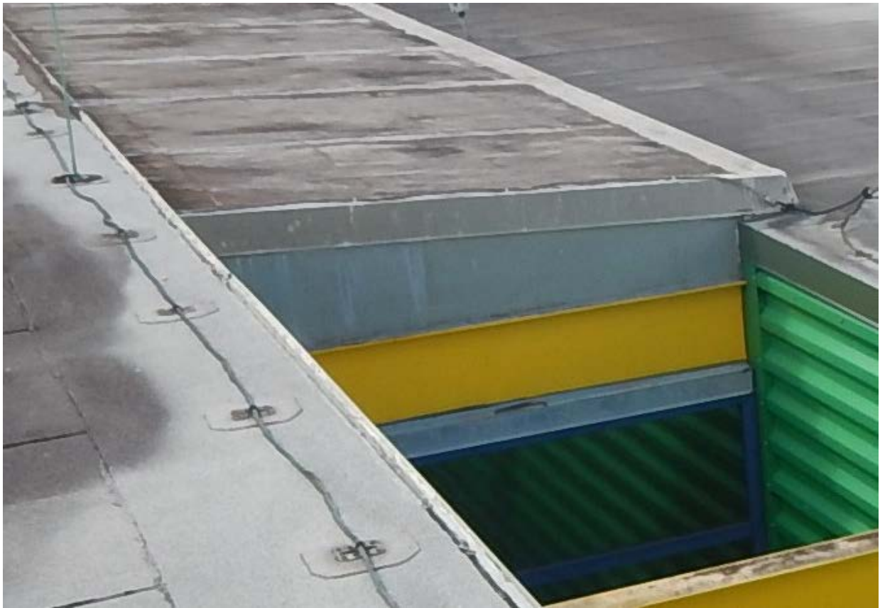
Photo 2 – 4" Insulation Core Sample at Upper Roof Area
