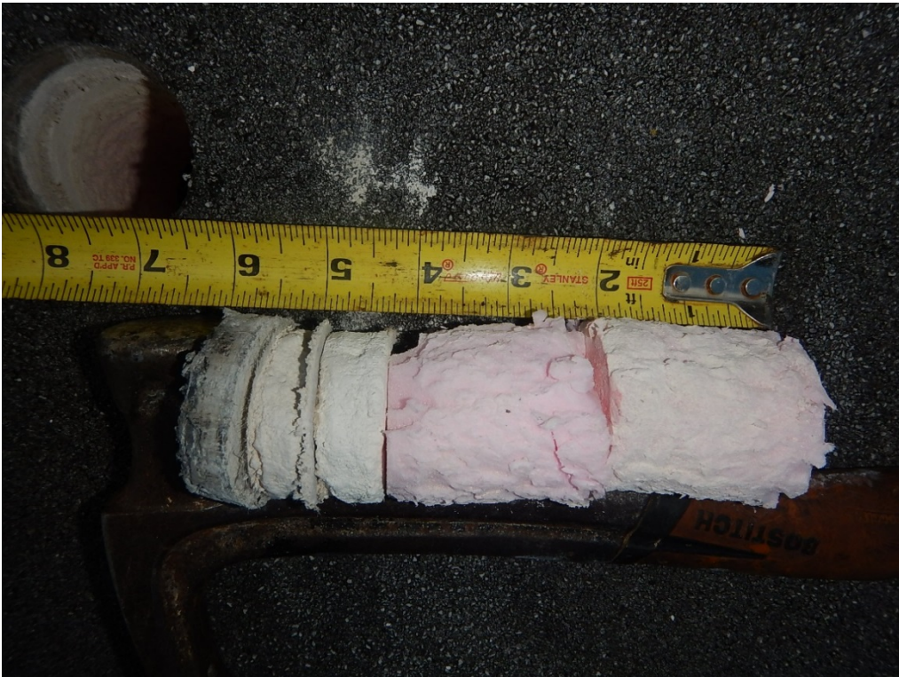
Photo 2 – 4" Insulation Core Sample at Upper Roof Area
