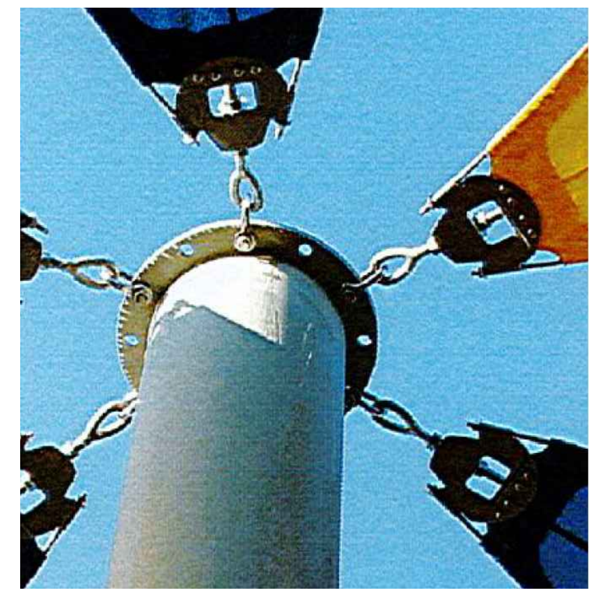
SAIL TENSIONER UNIT SHOWING QUICK RELEASE CONNECTION TO COLUMN
