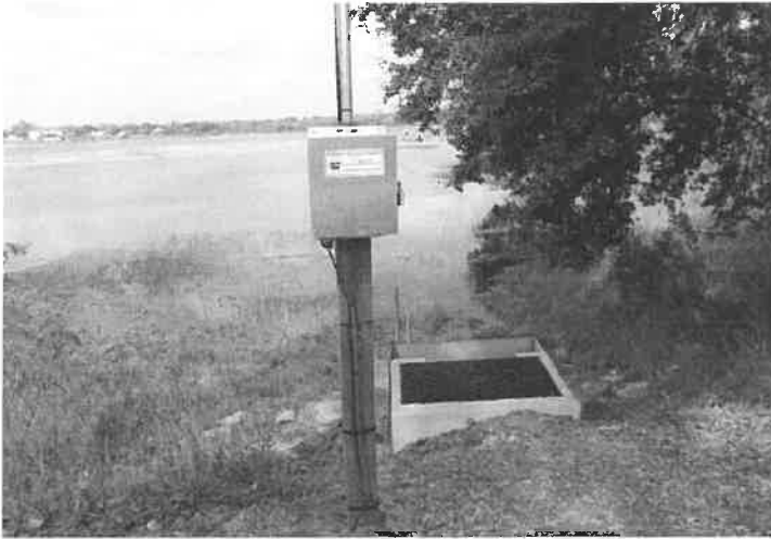
05 View of inflow structure located on Lake Hiawassee.
