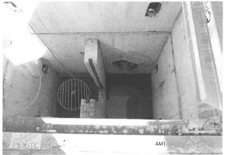
02. Interior view of well structure, showing inflow pipe from lake, concrete weir and wellhead with debris screen
