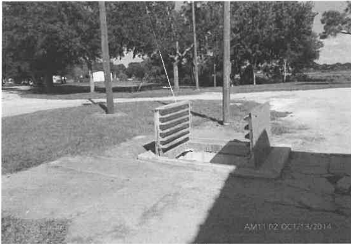
01. View of well structure with hatches open
