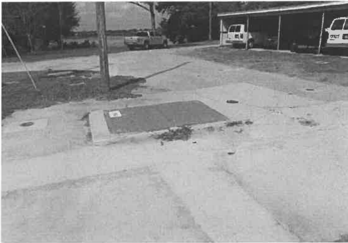
01. View of dainage well structure
