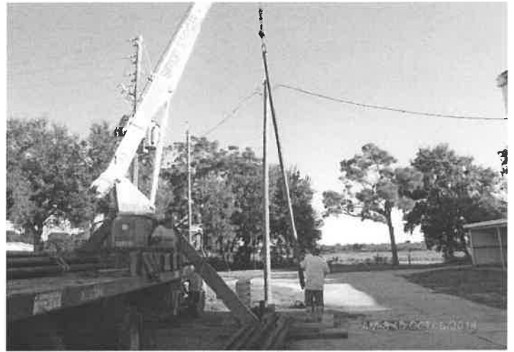
08. View of crew installing 4-inch dia steel pipe for cleaning well
