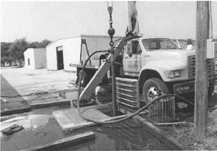
07. View of air-lift pipe set into position for well cleaning.
