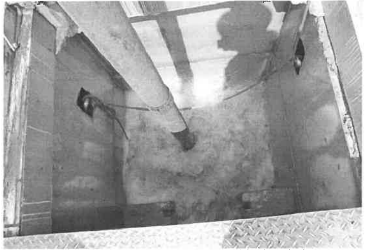
08. View of air-lift cleaning using the straight-air method.
