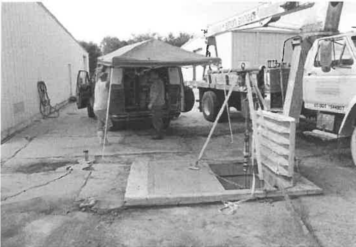
11. View of video logging equipment during logging
