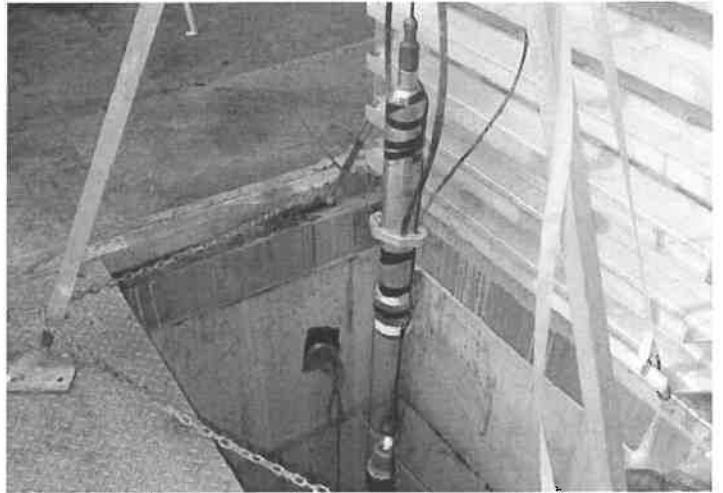
12. View of video camera being lowered into well
