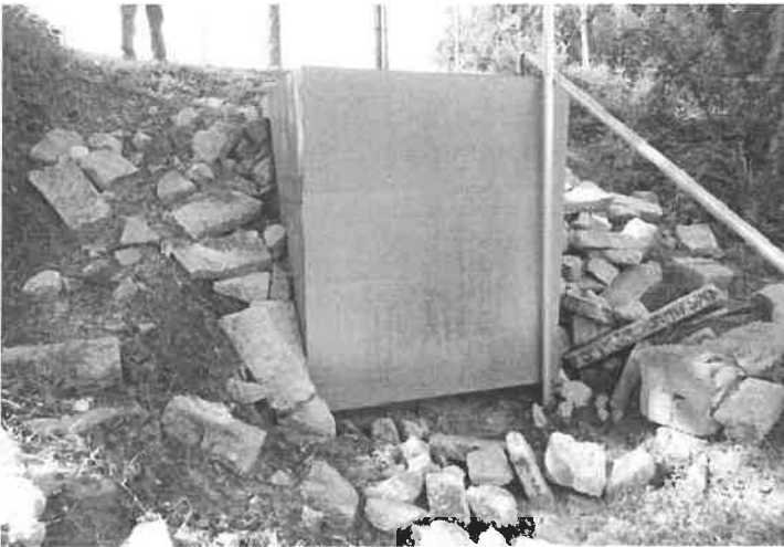
07. Additional view of skimmer and riprap
