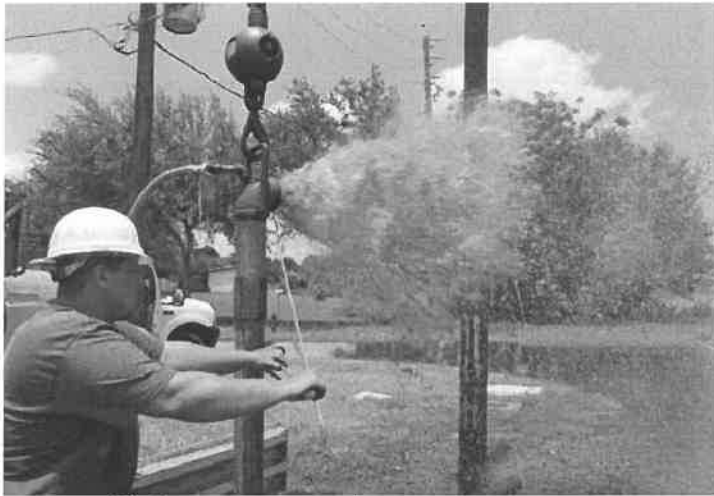
09. View of air-lift cleaning using the reverse-air method.
