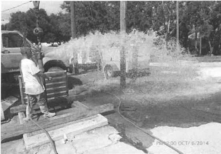
09. View of air lift discharge during well cleaning
