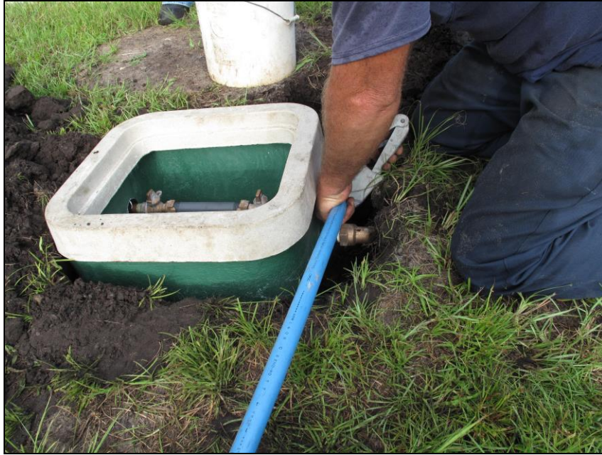
Figure 14. Cutting Polyethylene tubing
