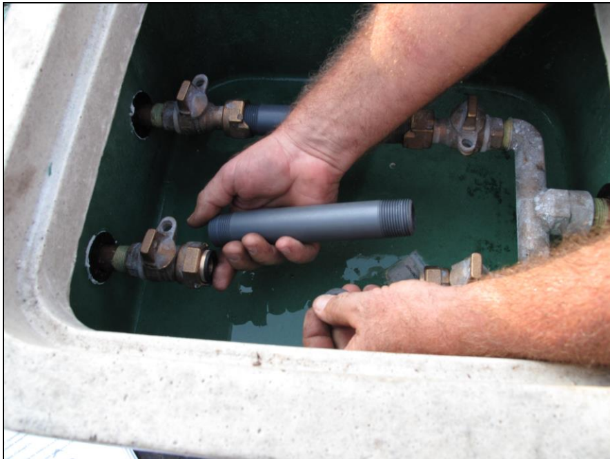
Figure 10. Removing the spacer
