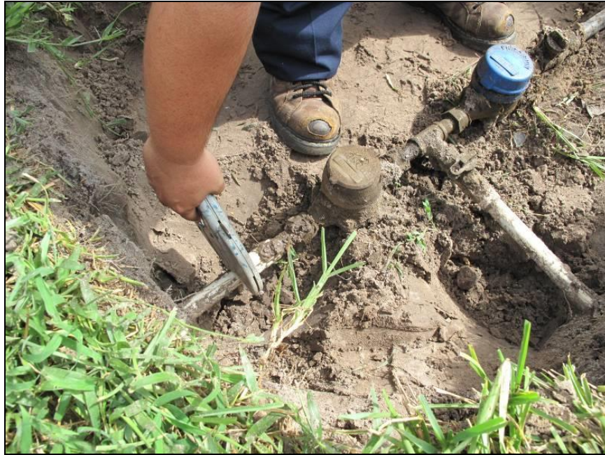
Figure 14. Cutting the house line
