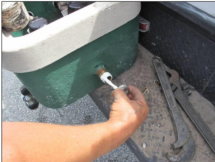
Figure 35. Applying joint compound to inlet thread
