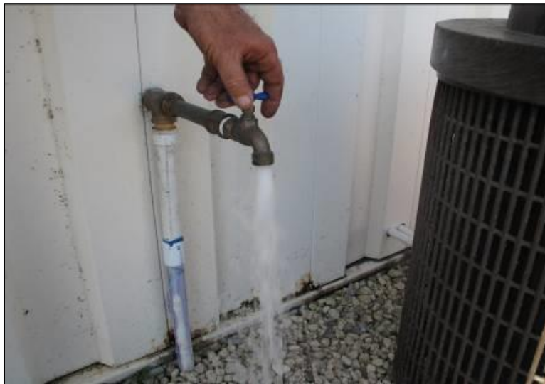
Figure 15. Flushing house line
