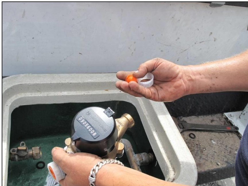
Figure 29. Preparing meter to be installed, removing end caps and thread protectors
