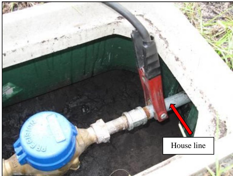
Figure C. The other end of jumper cable clamped on house line
