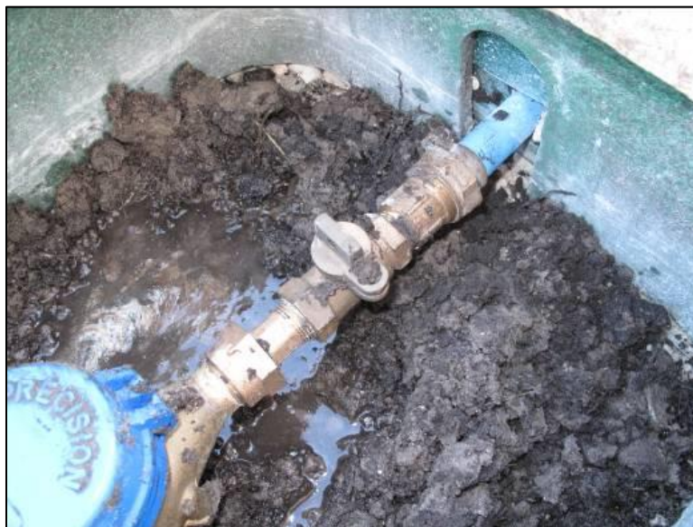
Figure 8. Closed curb stop
