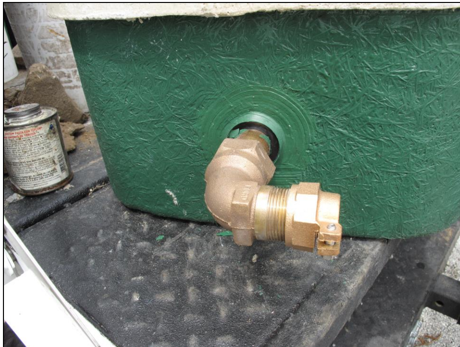
Figure 13. Thread by compression elbow
