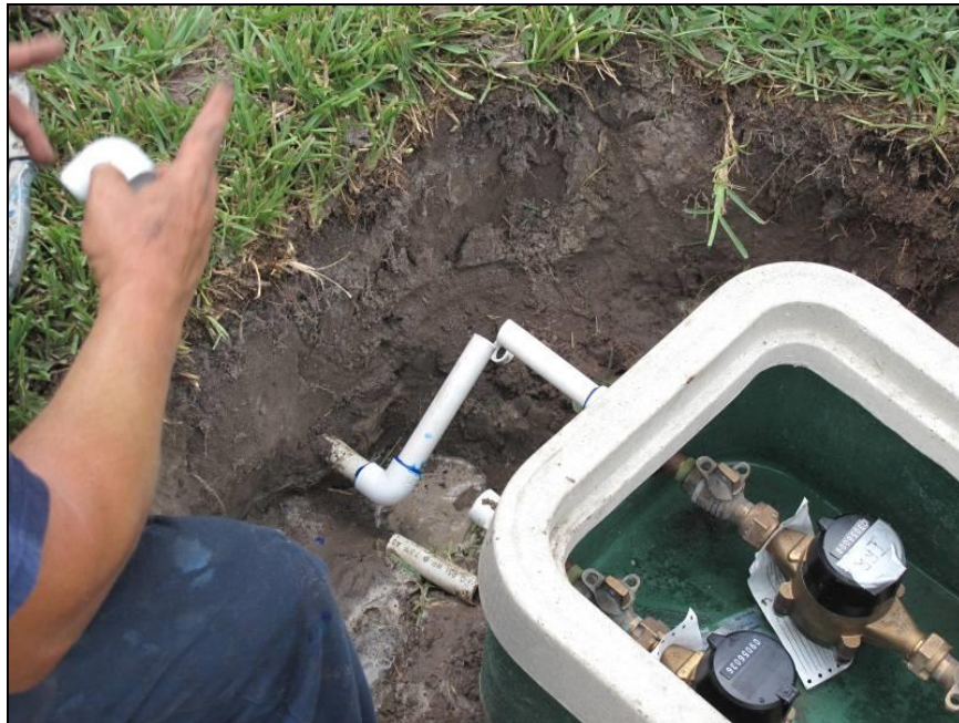
Figure 49. Aligning PVC
