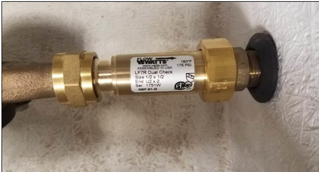
Figure 27. Backflow Preventer
