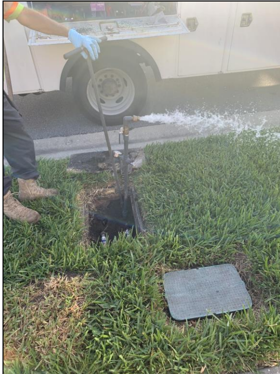
Figure 40. Flushing Service
