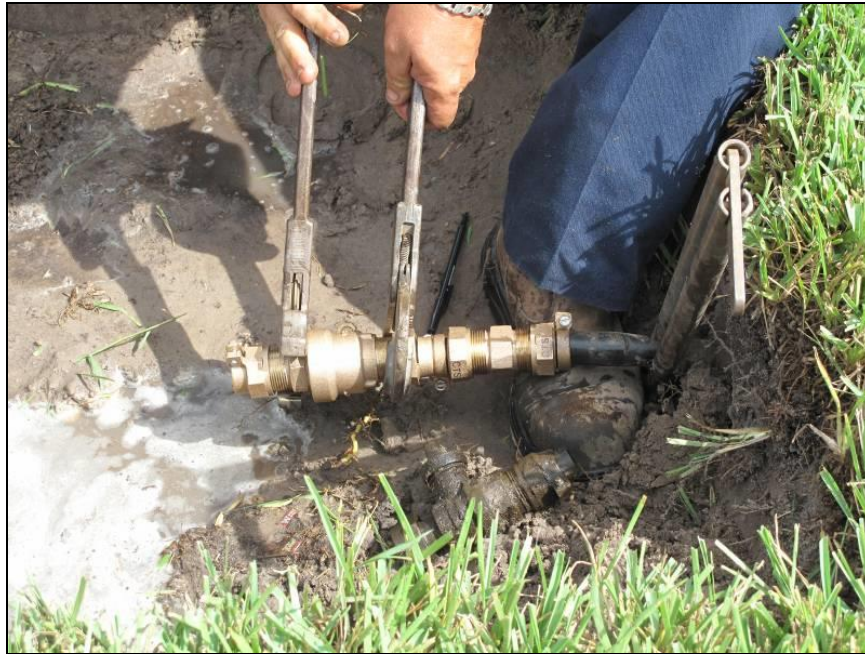
Figure 22. Tightening curb stop
