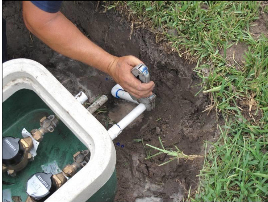
Figure 48. Cutting PVC
