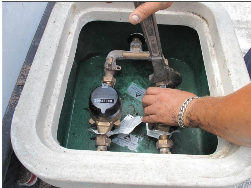
Figure 31. Tightening meters in new box
