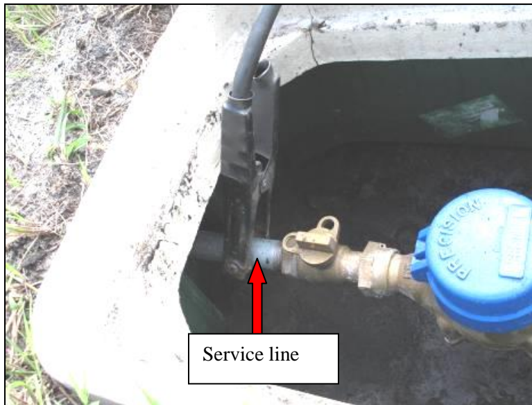
Figure 2. One end of jumper cable clamped on service line
