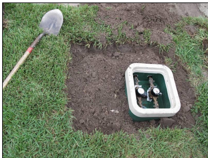
Figure 54. Backfilling and compacting
