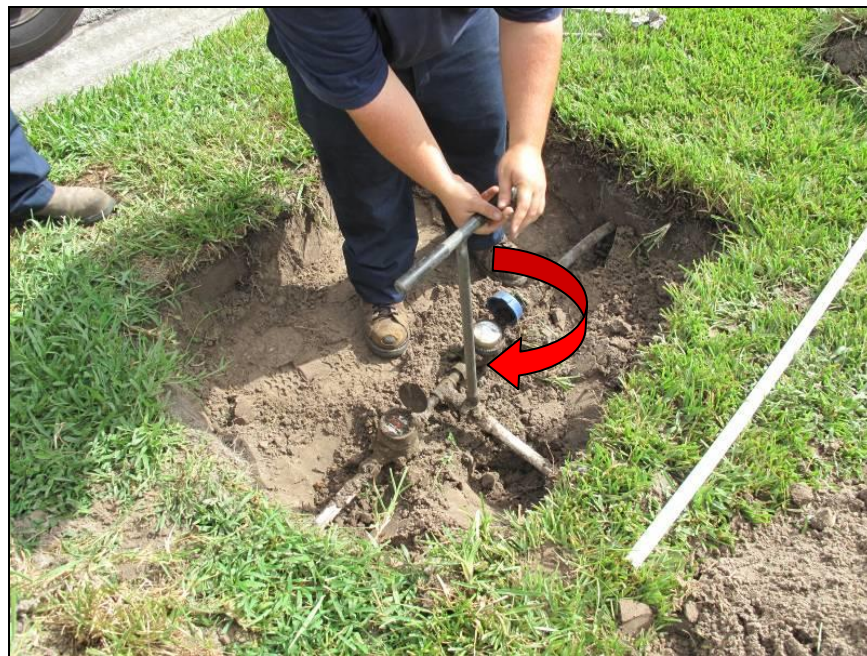
Figure 13. Closing additional curb stops
