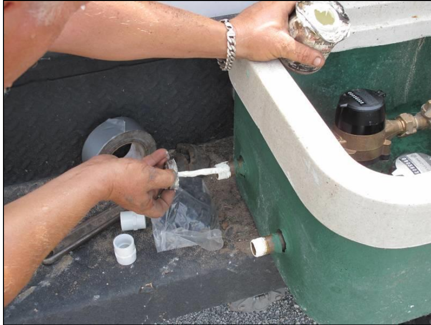
Figure 36. Applying joint compound to outlet threads
