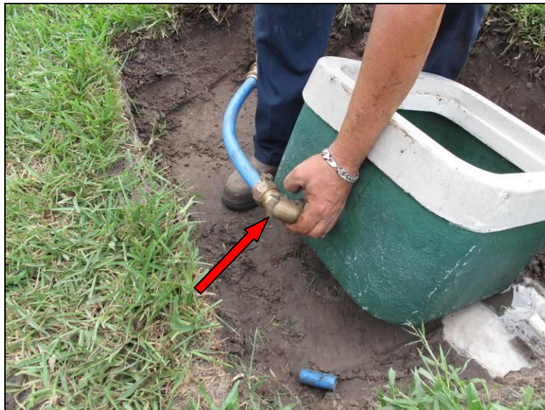
Figure 43. Poly into 90° thread by compression elbow
