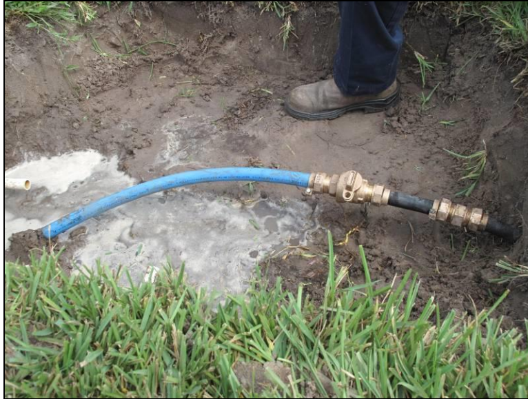
Figure 41. Polyethylene tubing installed in curb stop
