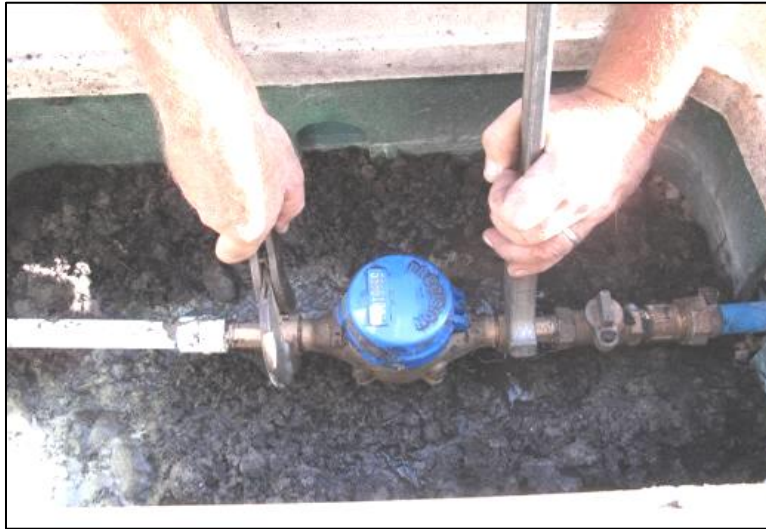
Figure 9. Removing meter using meter wrenches
