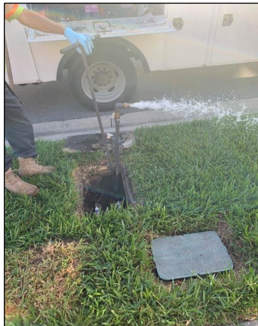
Figure 12. Flushing service
