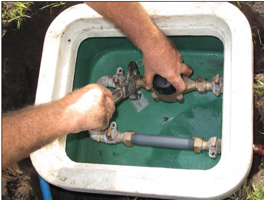
Figure 19: Tightening meter
