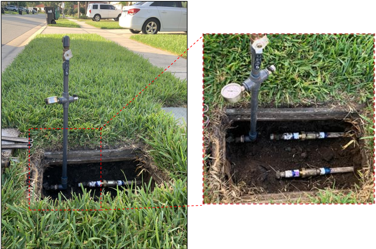
Figure 39. Standpipe Installed in Service Line
