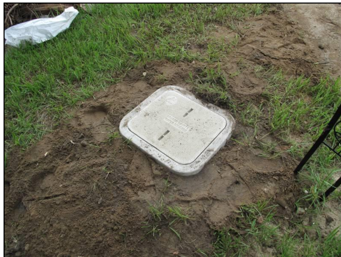
Figure 56. Completed job requiring a restoration request form
