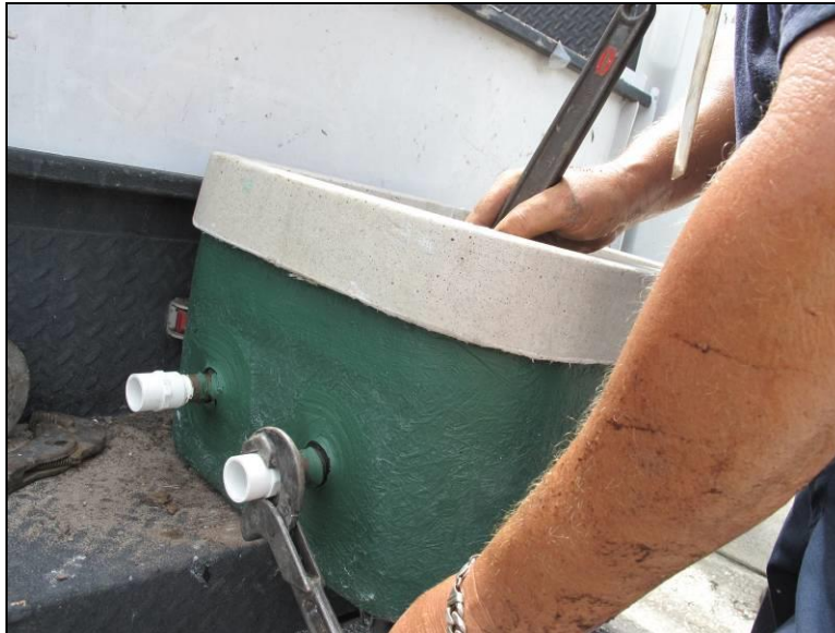
Figure 38. Tightening female adapters
