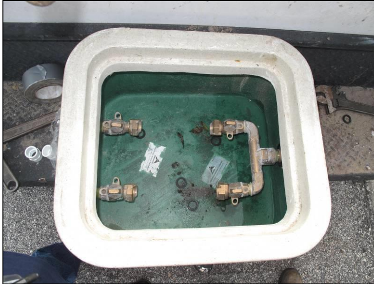
Figure 26. Spacers removed
