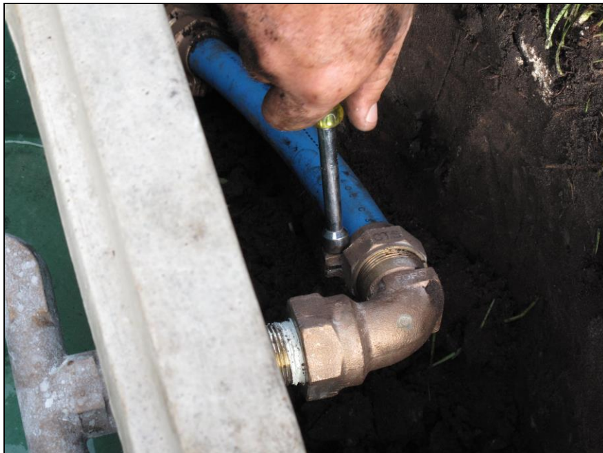
Figure 16. Tightening bolt on compression piece
