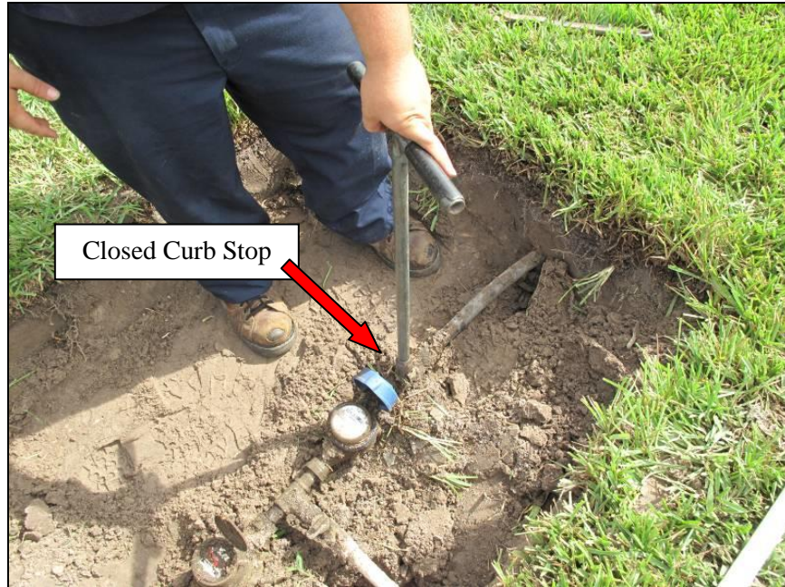
Figure 12. Closed Curb Stop
