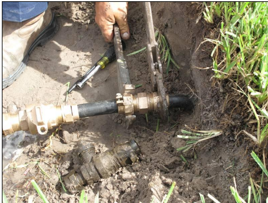
Figure 23. Tightening compression coupling
