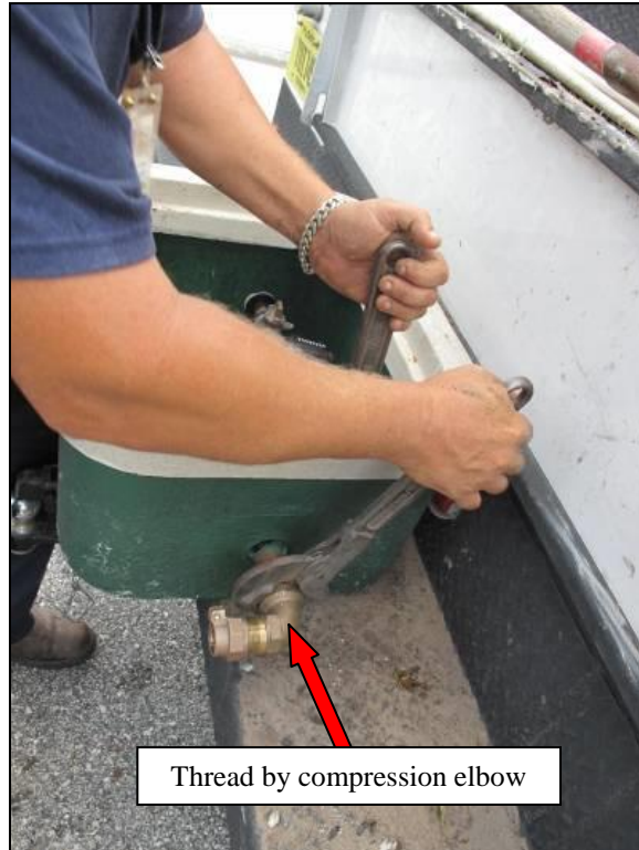
Figure 37. Thread by compression elbow and tightening using two meter wrenches
