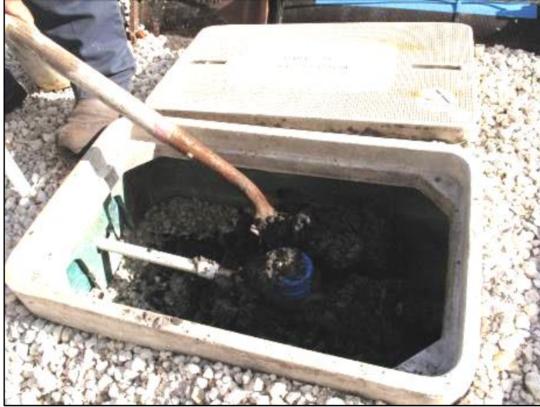
Figure 3. Cleaning out meter box
