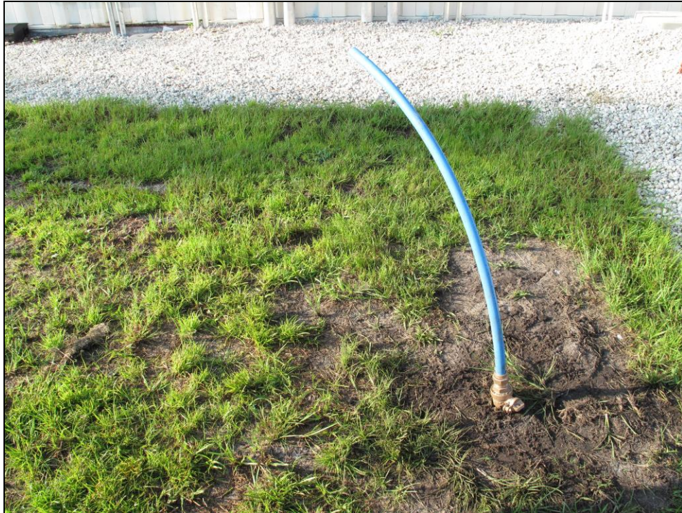
Figure 2. Water service location identified by service line above grade
