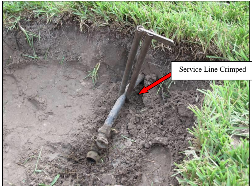
Figure 18. Service line crimped
