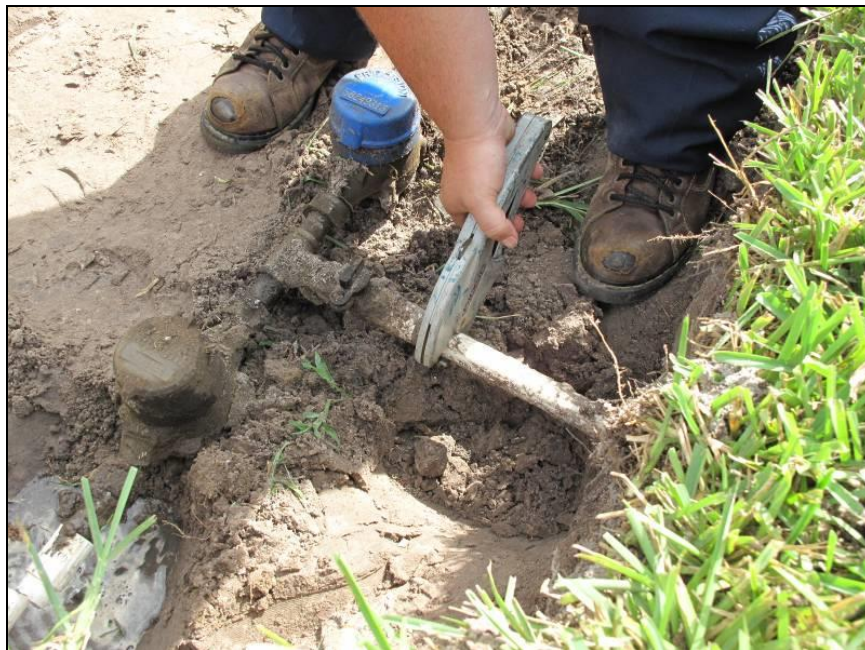
Figure 15. Cutting the irrigation line
