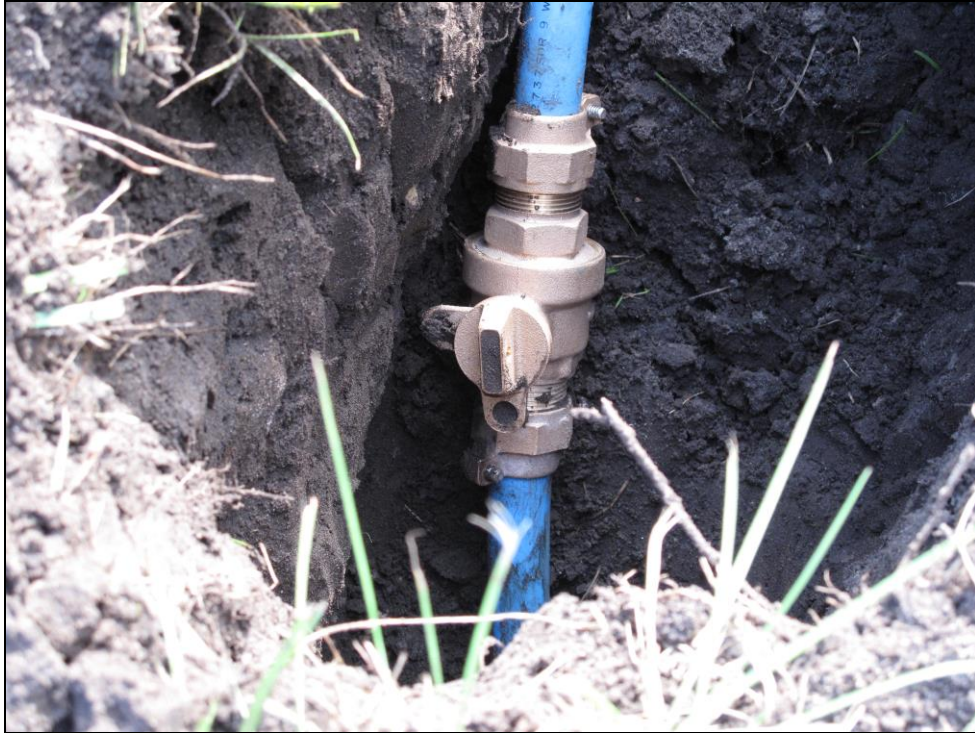
Figure 18. Opened Curb Stop
