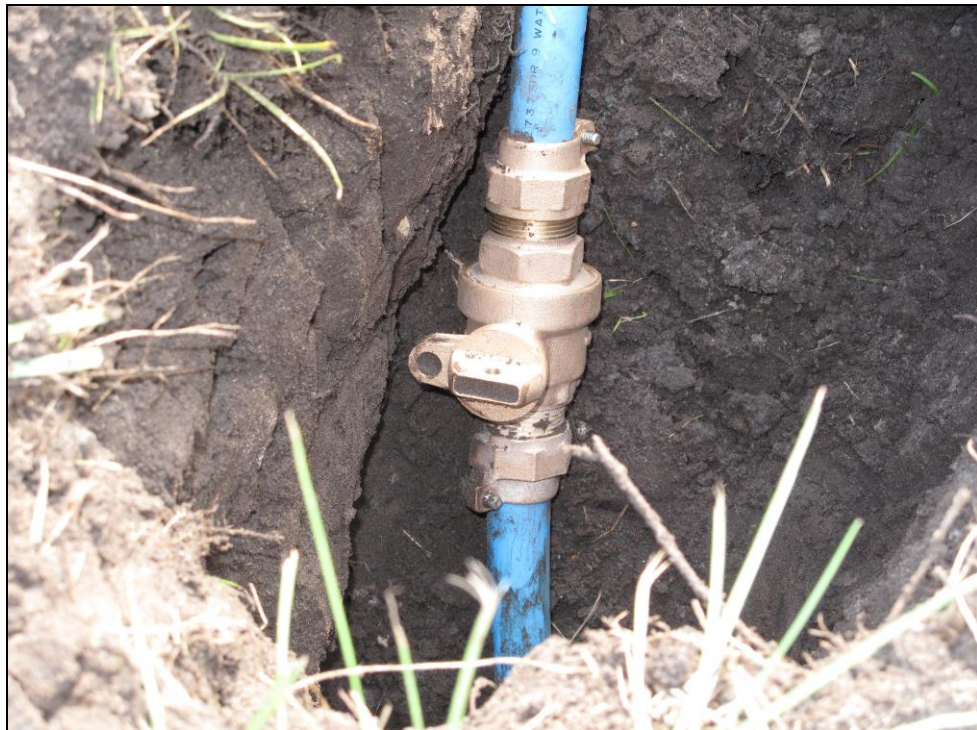
Figure 17. Closed Curb Stop
