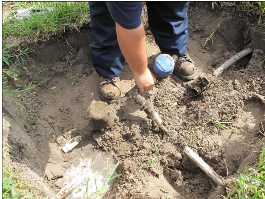
Figure 17. Meters Removed
