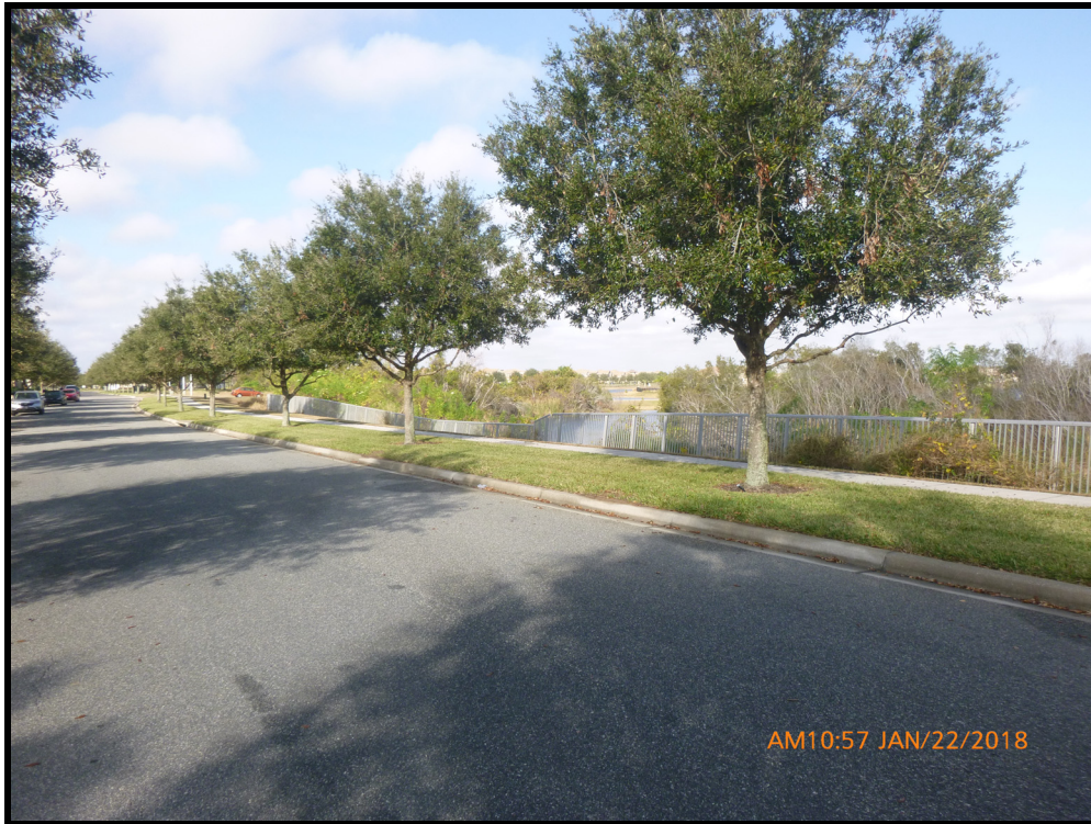
Exhibit 11. View of Retaining Wall Fence From Porter Road Looking NW (1/22/18)
