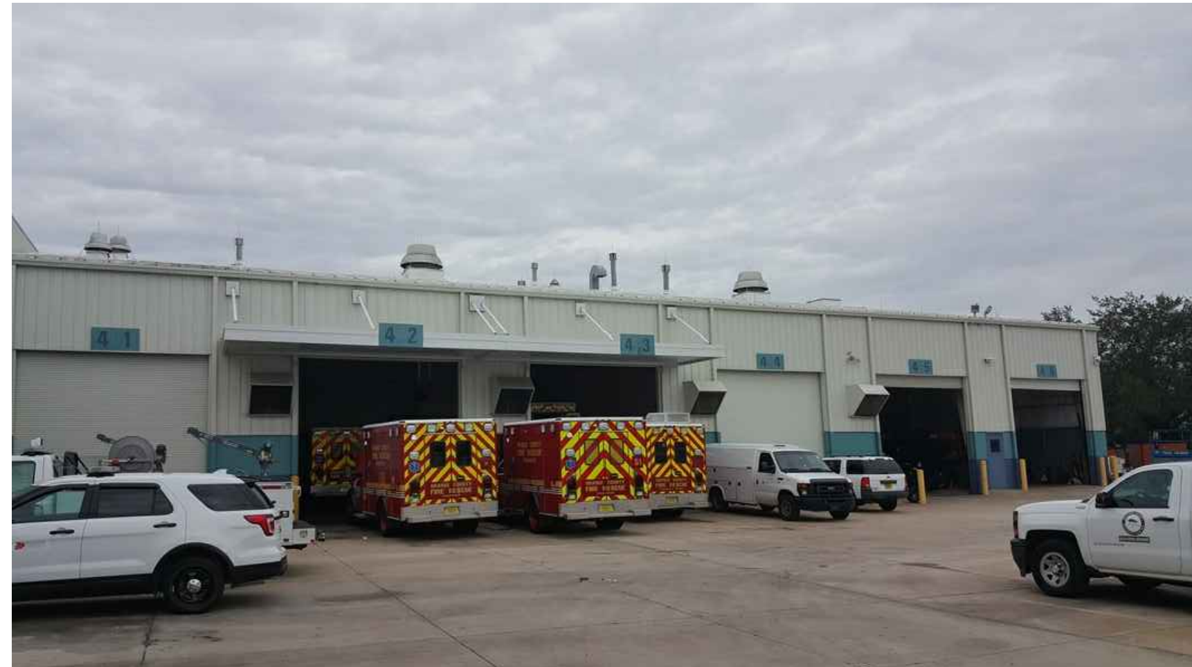
OVERVIEW AT EXISTING BUILDING CANOPY 1 SCALE: N.T.S.
