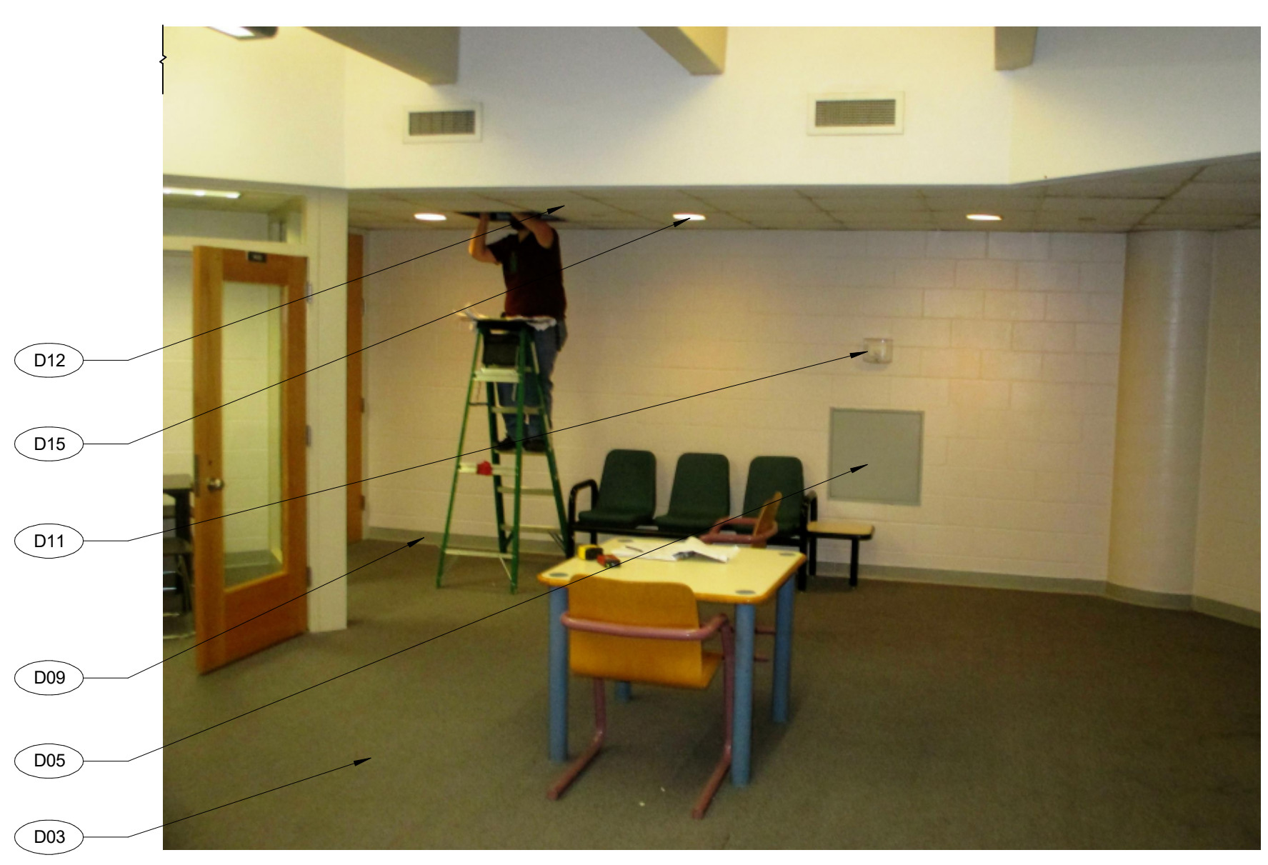
2 AD103 EXISTING PHOTO AT LEVEL 3 VISITATION (352) CHASE WALL SCALE: 1/4" = 1'-0"
