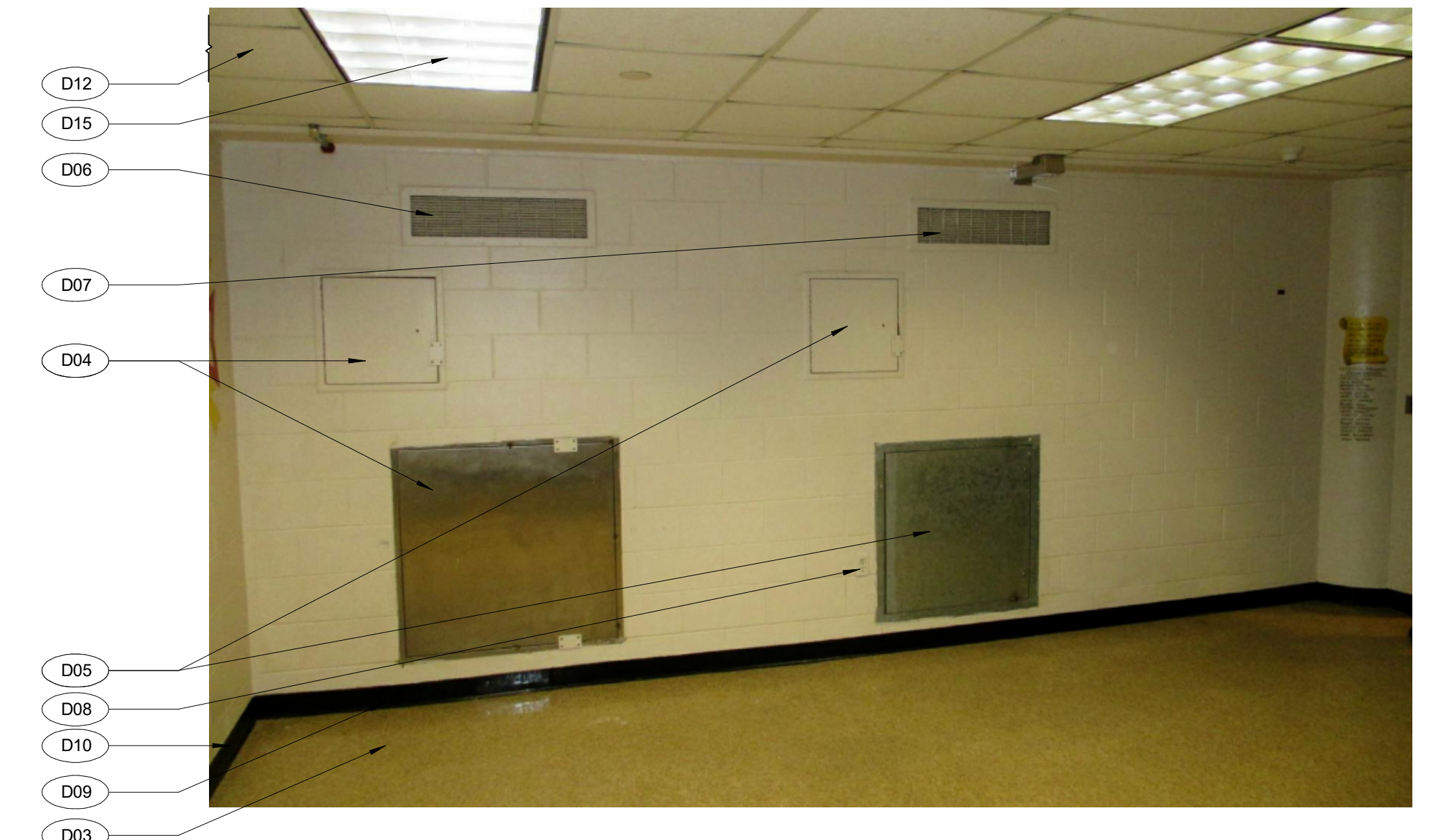
6 AD102 EXISTING PHOTO AT LEVEL 2 CLASSROOM "C" CHASE WALL SCALE: 1/4" = 1'-0"
