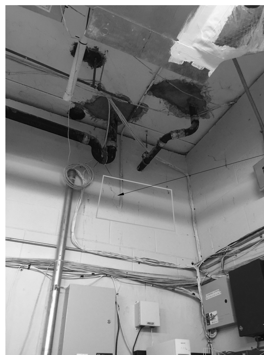
RELOCATE EXISTING CONDUIT TO ACCOMMODATE NEW DUCT
