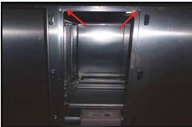
Figure 5. Door header and jambs
