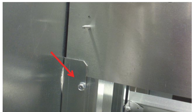
Figure 8. Screws internal to the wall
