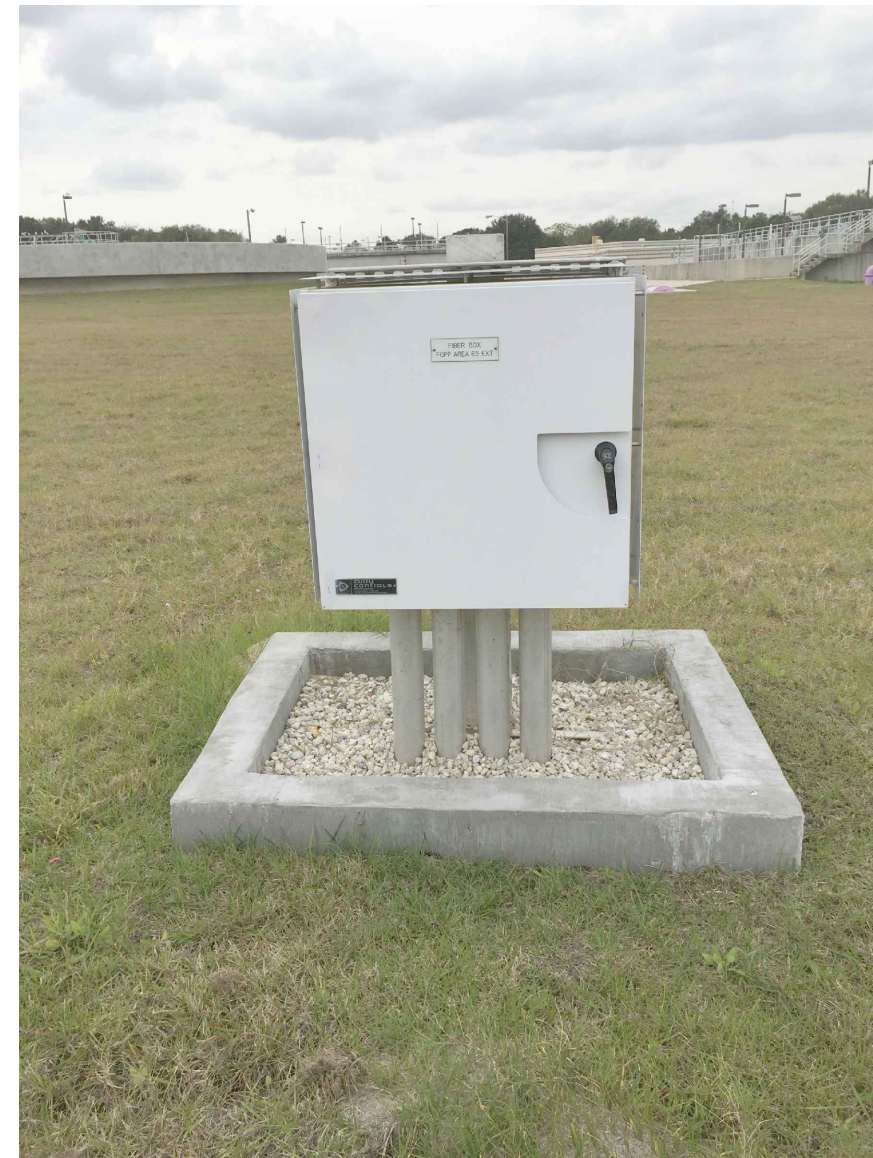
1 E-2 FIGURE NO. 1 AREA 65 FOPP EXT FIBER PATCH PANEL SCALE: N.T.S.
