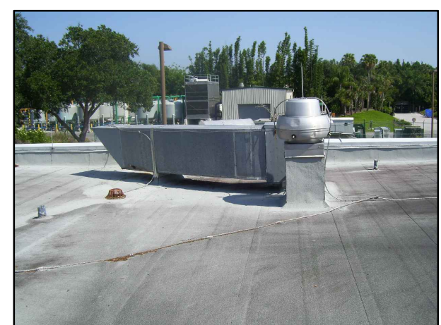
KITCHEN HOOD SUPPLY & EXHAUST FAN
