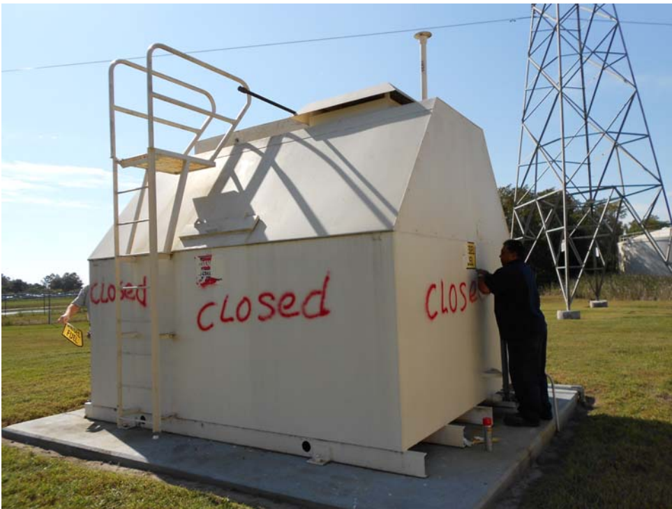
Photo of AST after being decommissioned / closed 11/1/12
