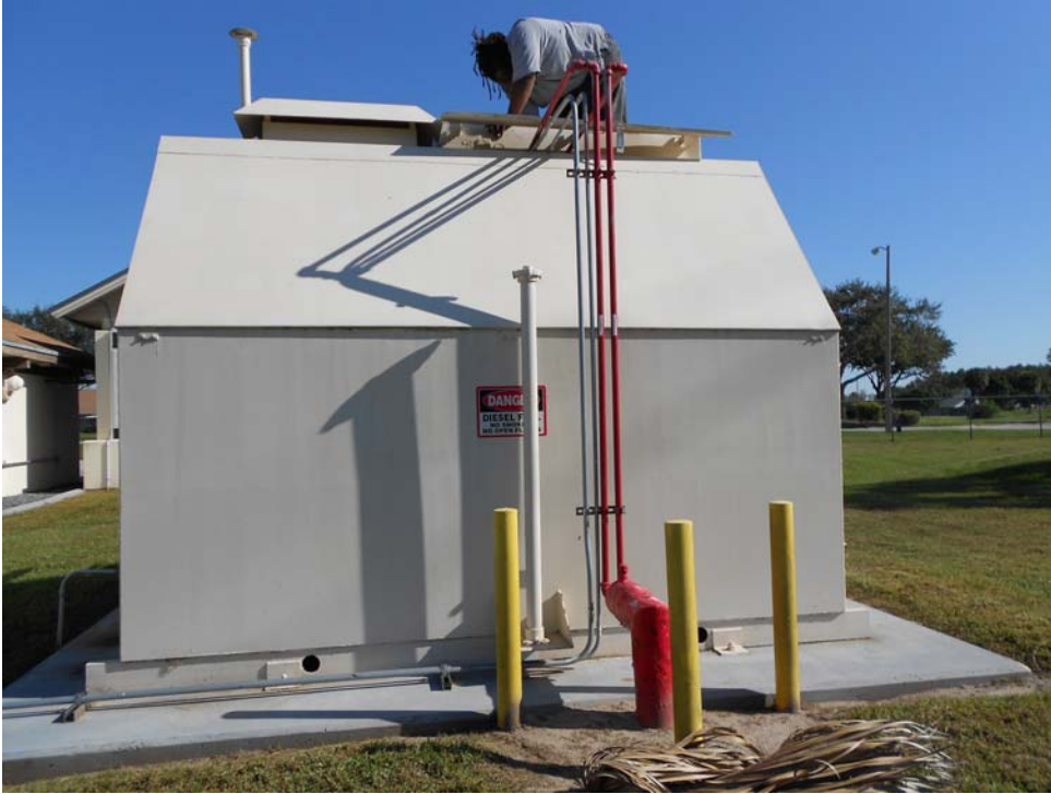
Photo of tank during decommissioning process 10/31/12
