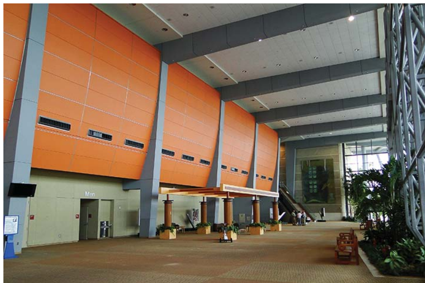
Orange panels cover the curved wall and are separated by columns.
