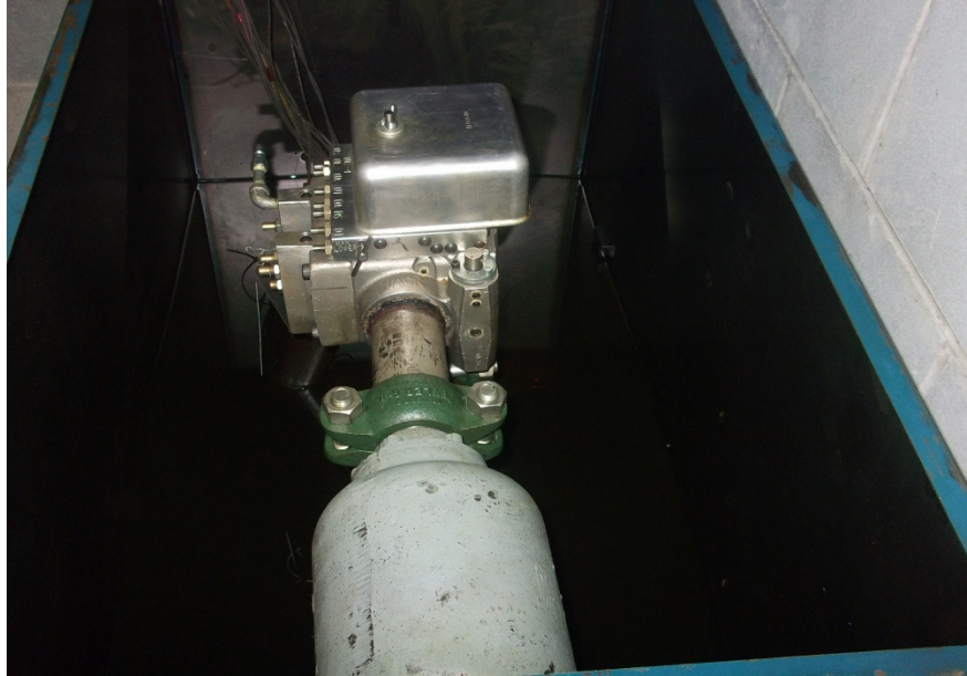
Above: Submersible pumping unit consists of components that are no longer manufactured for direct replacement.
