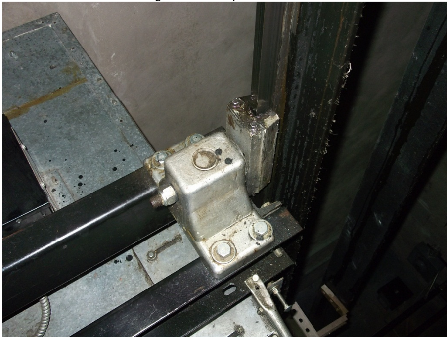
Above: Car top equipment and car side door equipment to be replaced; to include, door operator, clutch w/restrictor, inspection station, and code compliant escape hatch. Below: Slide guides to be replaced with newer inserts.
