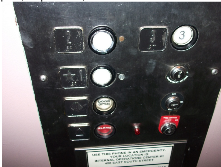
Above & Below: Car operating panel will be replaced in full, offering a hands free emergency phone, LED pushbuttons, vandal resistance materials and structure.
