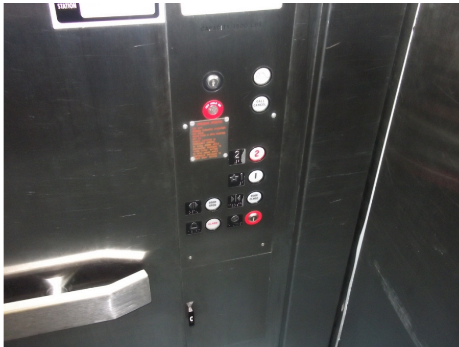
Below: Car Operating Panel will be replaced with LED, Vandal Resistant buttons and a hands free phone.
