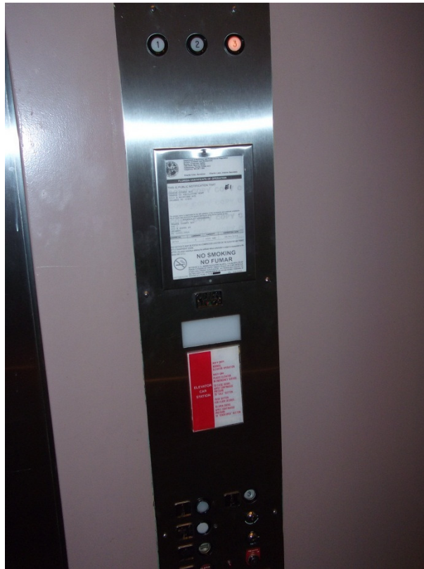
Above & Below: Car operating panel will be replaced in full, offering a hands free emergency phone, LED pushbuttons, vandal resistance materials and structure.
