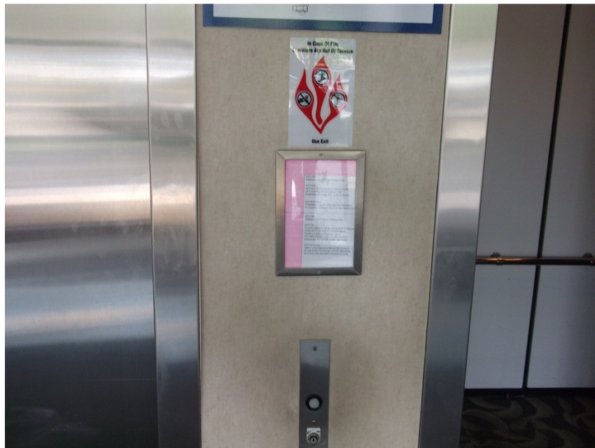
Above: Shaft requires ventilation and smoke head that is accessible from top lobby floor Below: Main lobby floor to have hall station with signage and fire service instructions engraved, dual position indicators and Regional Florida Fire Key Switch.
