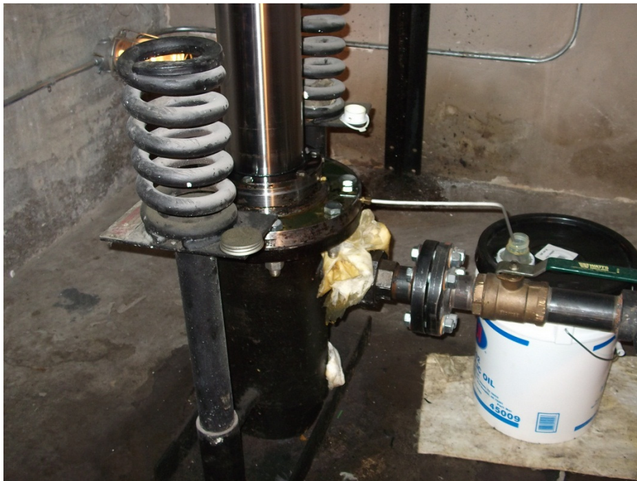
Above: General Contractor responsible for ensuring sump pump in pit meets local plumbing code Below: Jack packing requires replacement immediately, spring buggers to be retained, pit painted
