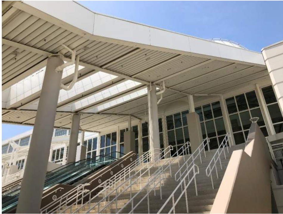
Photo #4 – South Concourse Canopy
