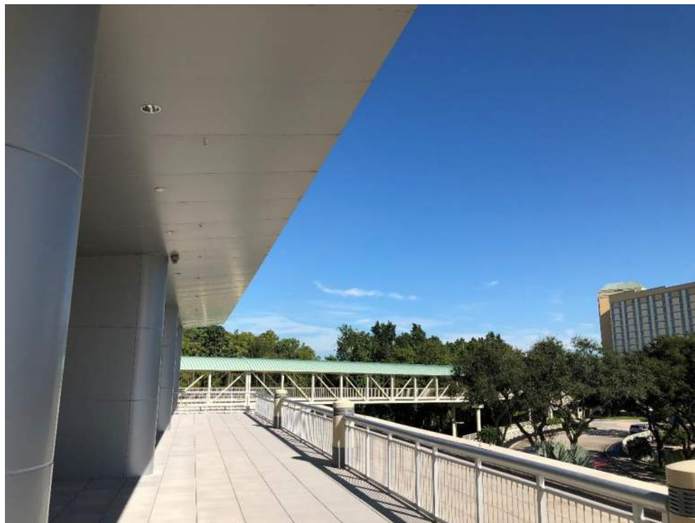
Photo #15 – Exterior Sunburst Balcony
