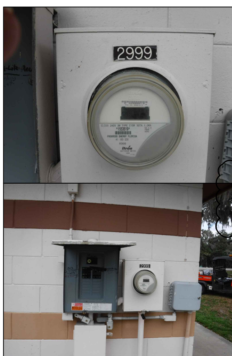
EXISTING NEMA 3R ELECTRICAL PANEL "c" EXISTING METER No. 1553519.
