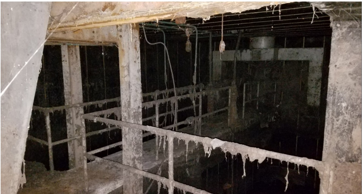
10 Middle level of screen structure
