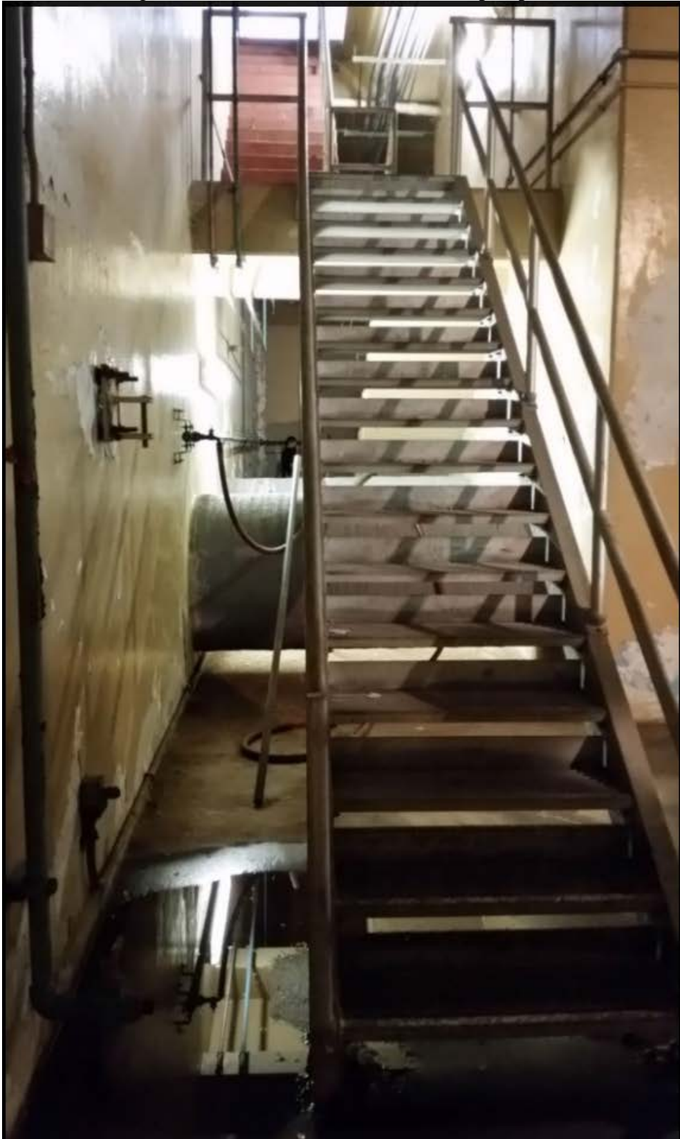
7. Looking south from the east side of the north pump room
