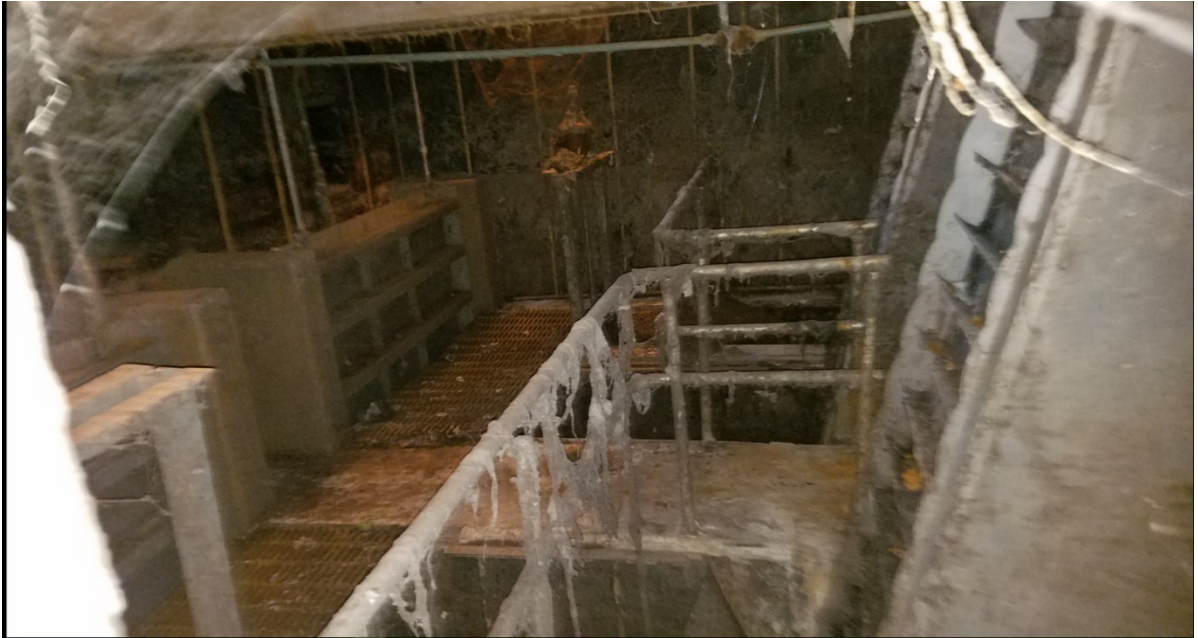
9. Middle level of screen structure
