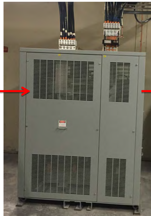
Fig. 2.2 Typical OUC 750Kva
