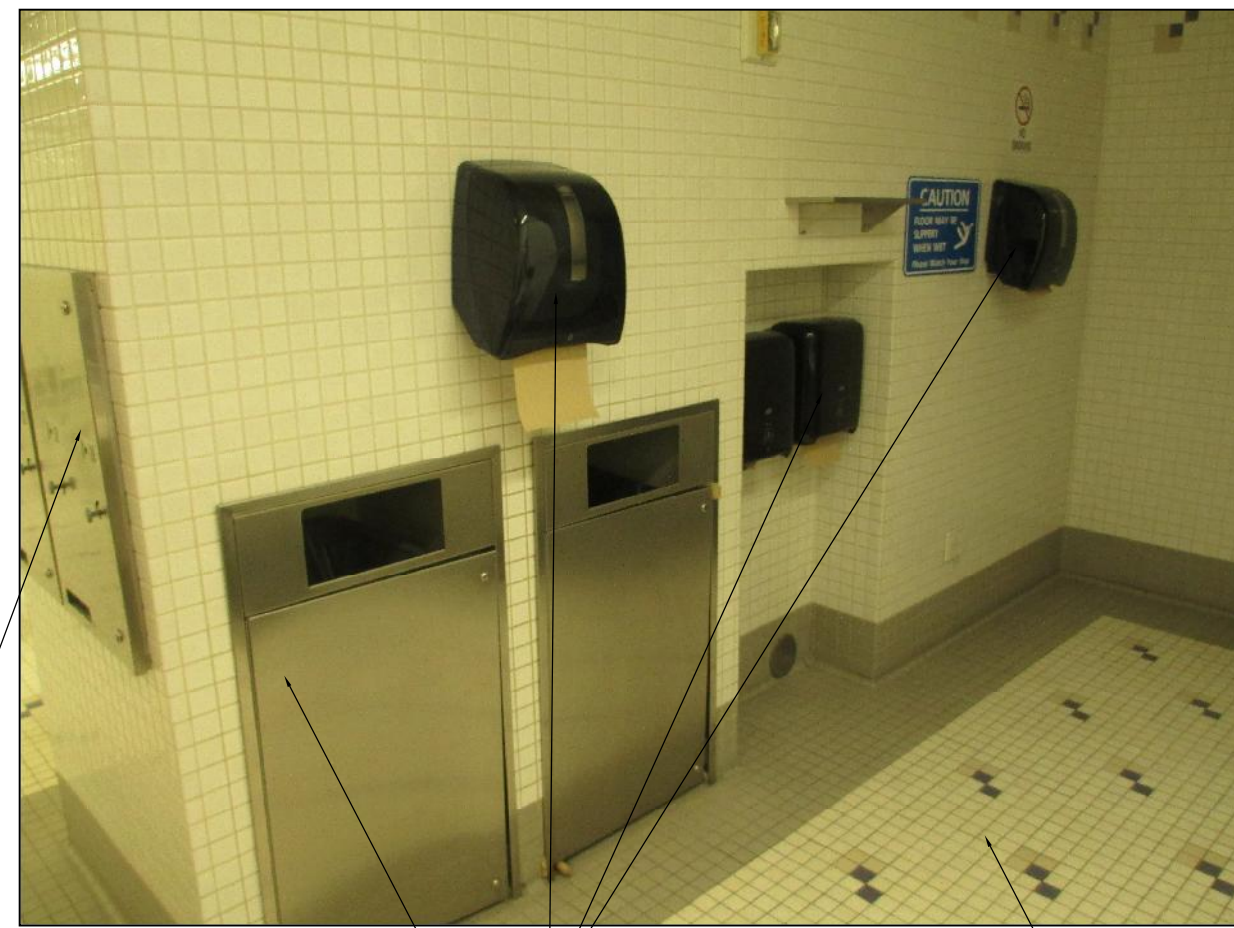
E3 AD601 CONCOURSE D - LEVEL 2 EXISTING IMAGES - ROOMS 259/260 scale: NTS
