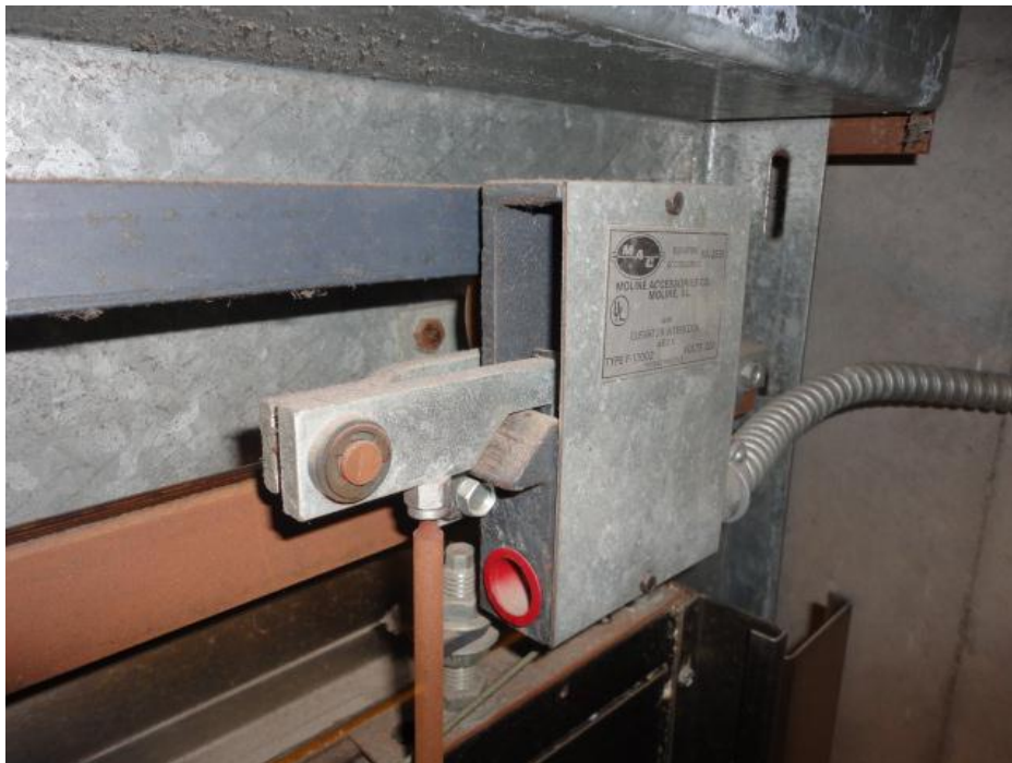
The hoistway door unlocking devices (top picture) and interlocks (bottom picture) will be replaced with new and compatible with new door operation.
