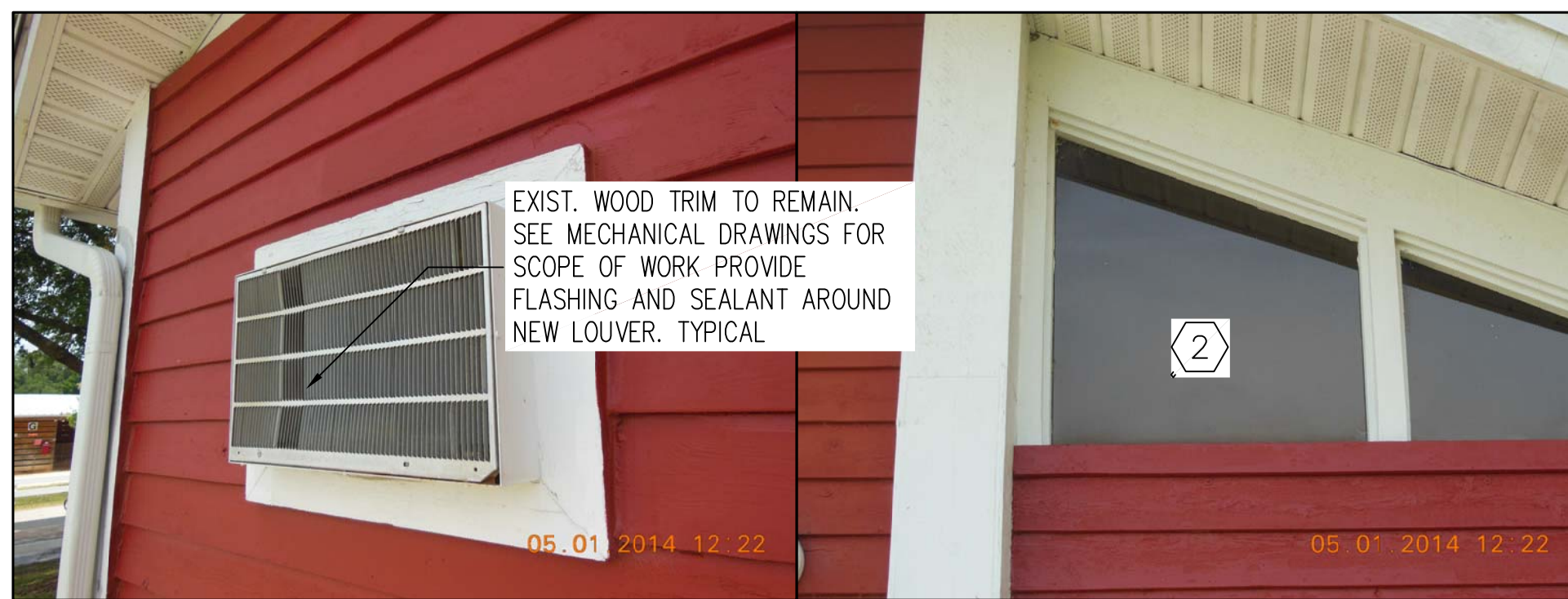
6 PHOTO - EXTERIOR AD100
