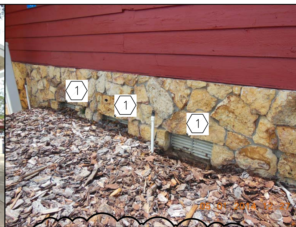
3 PHOTO - EXTERIOR AD100
