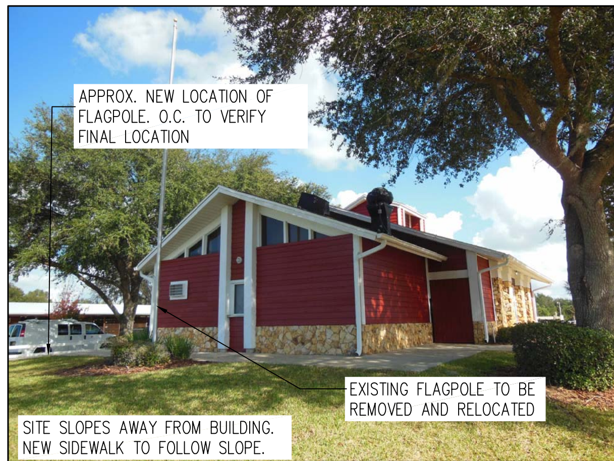
15 PHOTO - EXTERIOR AD100
