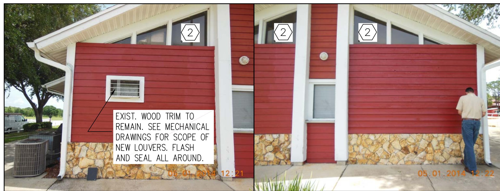
1 PHOTO - EXTERIOR AD100
