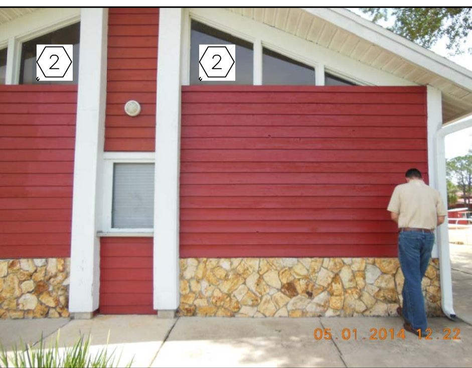
2 PHOTO - EXTERIOR AD100
