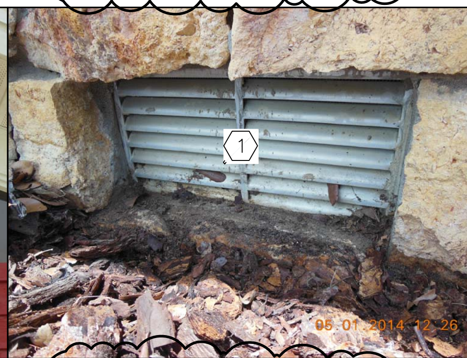
8 PHOTO - EXTERIOR AD100
