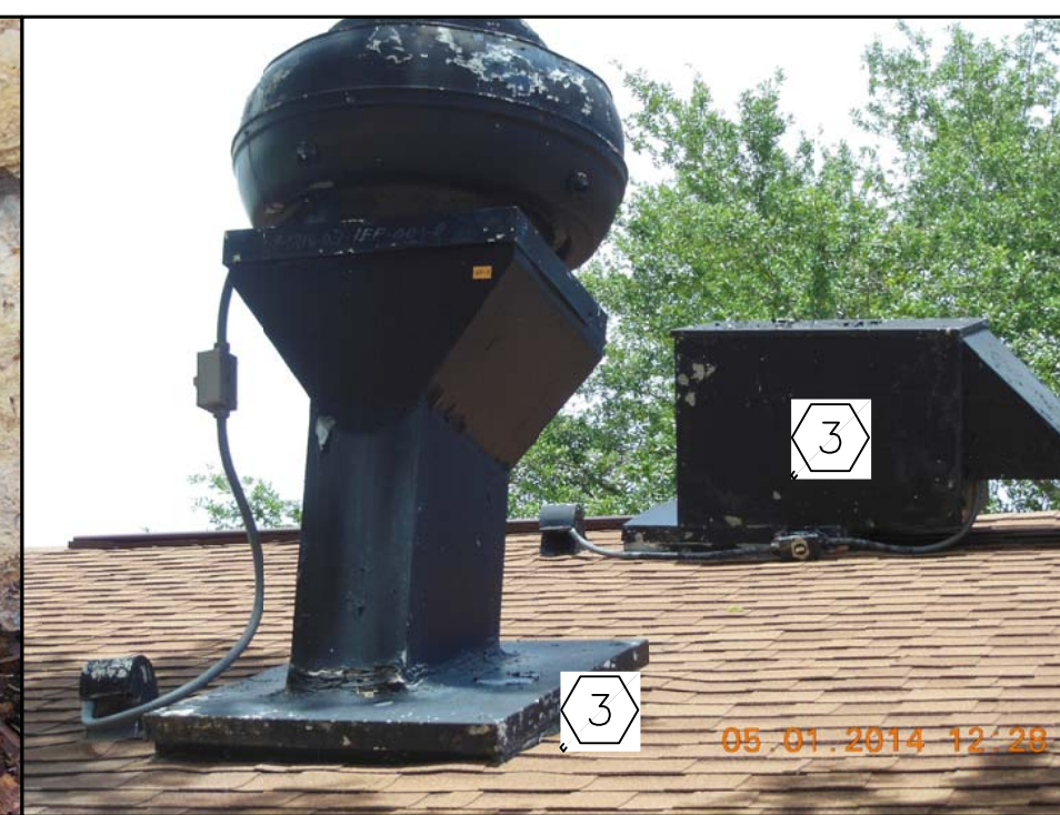
9 PHOTO - EXTERIOR AD100
