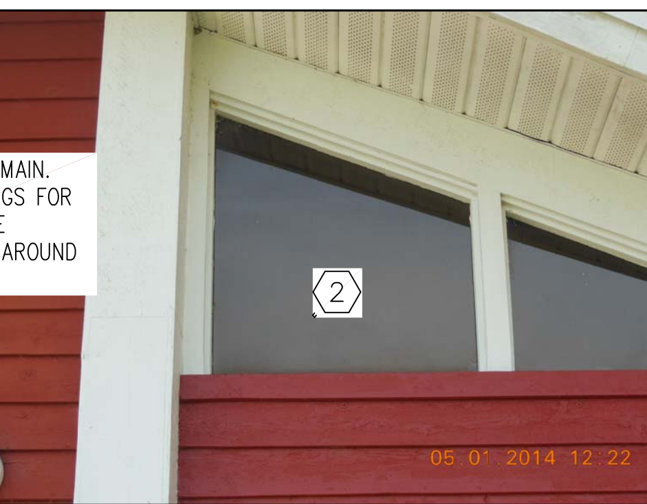
7 PHOTO - EXTERIOR AD100
