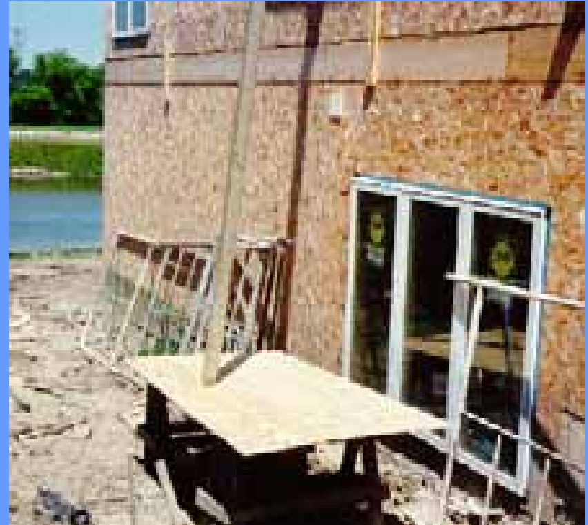
Expanded view of scaffold leg footing.
