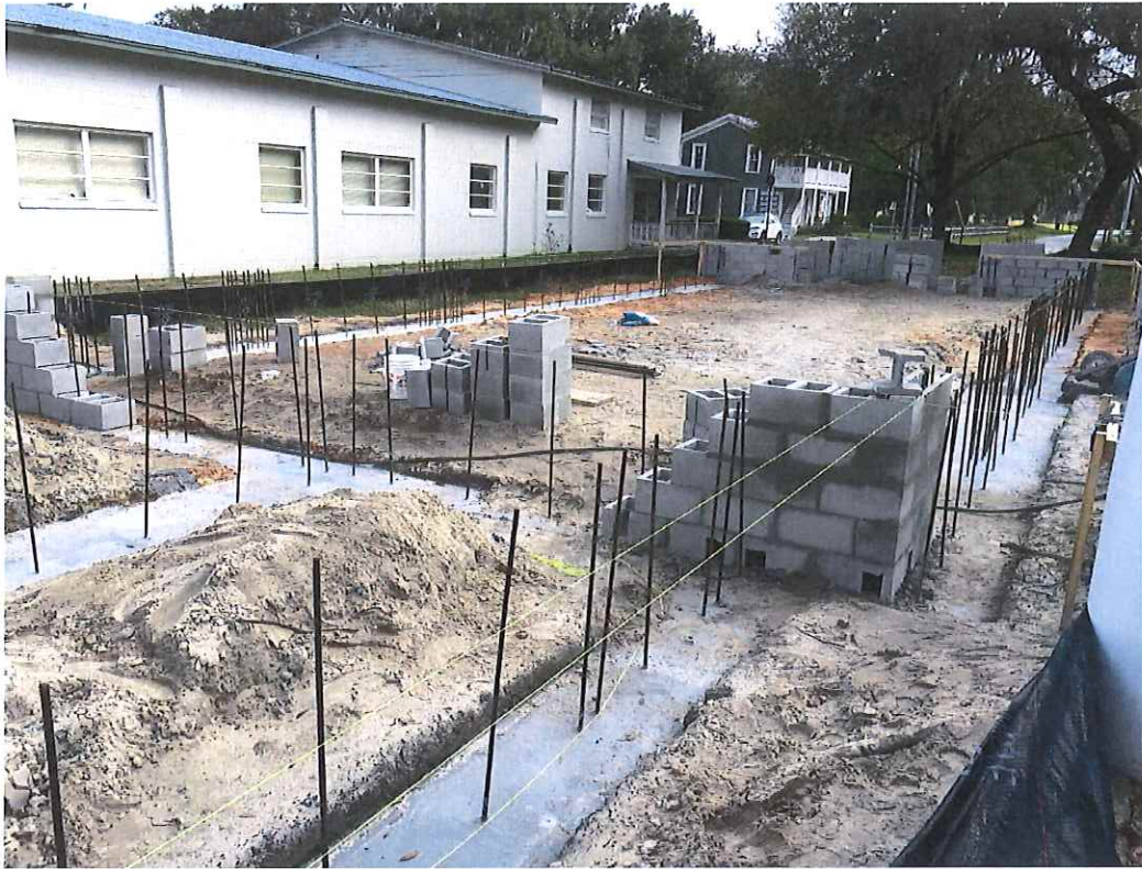
The footers are in place and stem walls begin to take shape. – February 7, 2019.
